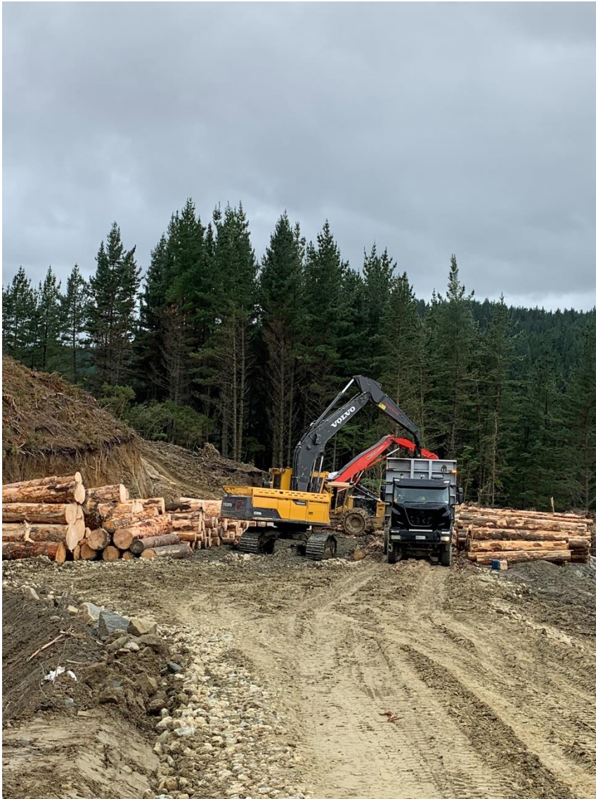
Photo 6: Log 16 working on the McCoy Road / Gray Road junction.
