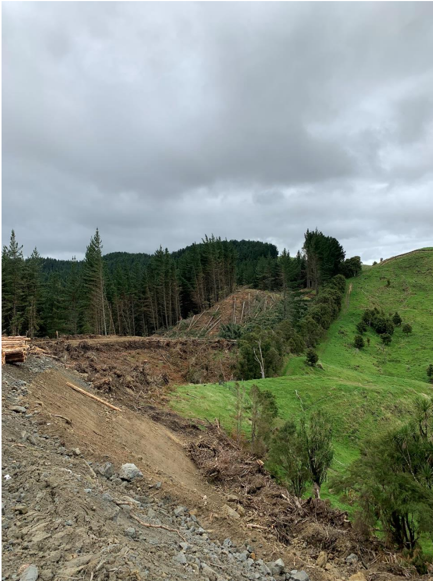
Photo 7: Log 16 working on the McCoy Road / Gray Road junction.
