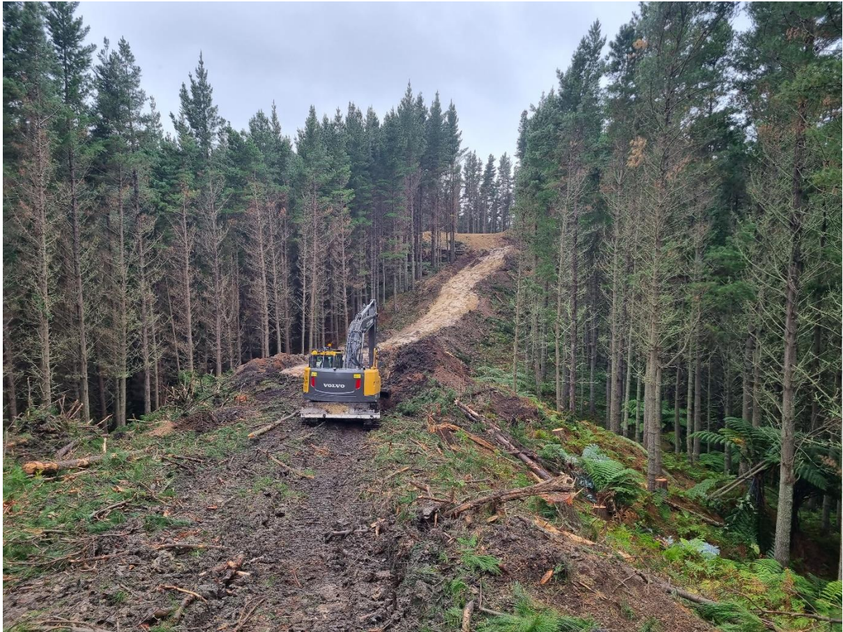
Photo 5: Road formation beginning from Landing 35 to 37.
