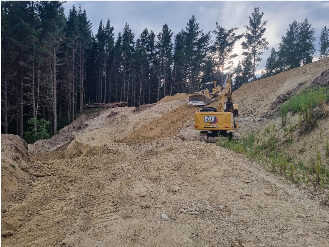
Photo 1: Earthworks underway to form a road to join Landing 36 to Kiwi Road.
