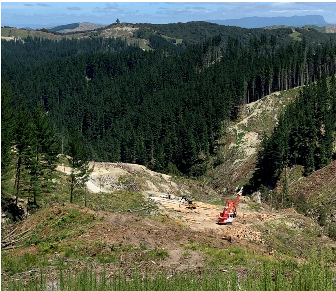
Photo 2: Log 27 working off Landing 206.
