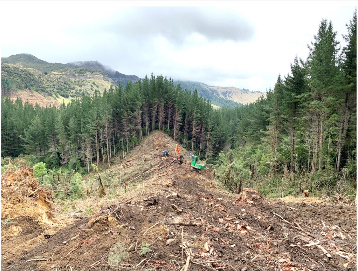
Ground-based harvesting off the ridge back to Landing 67.
