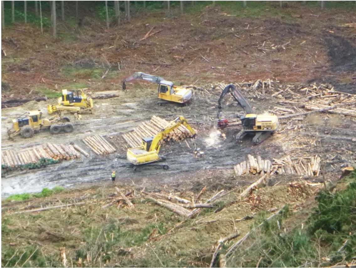
Photo 1: Log 15 operating on Landing 4 at the current end of Smith Road, roadlining in Setting 500.
