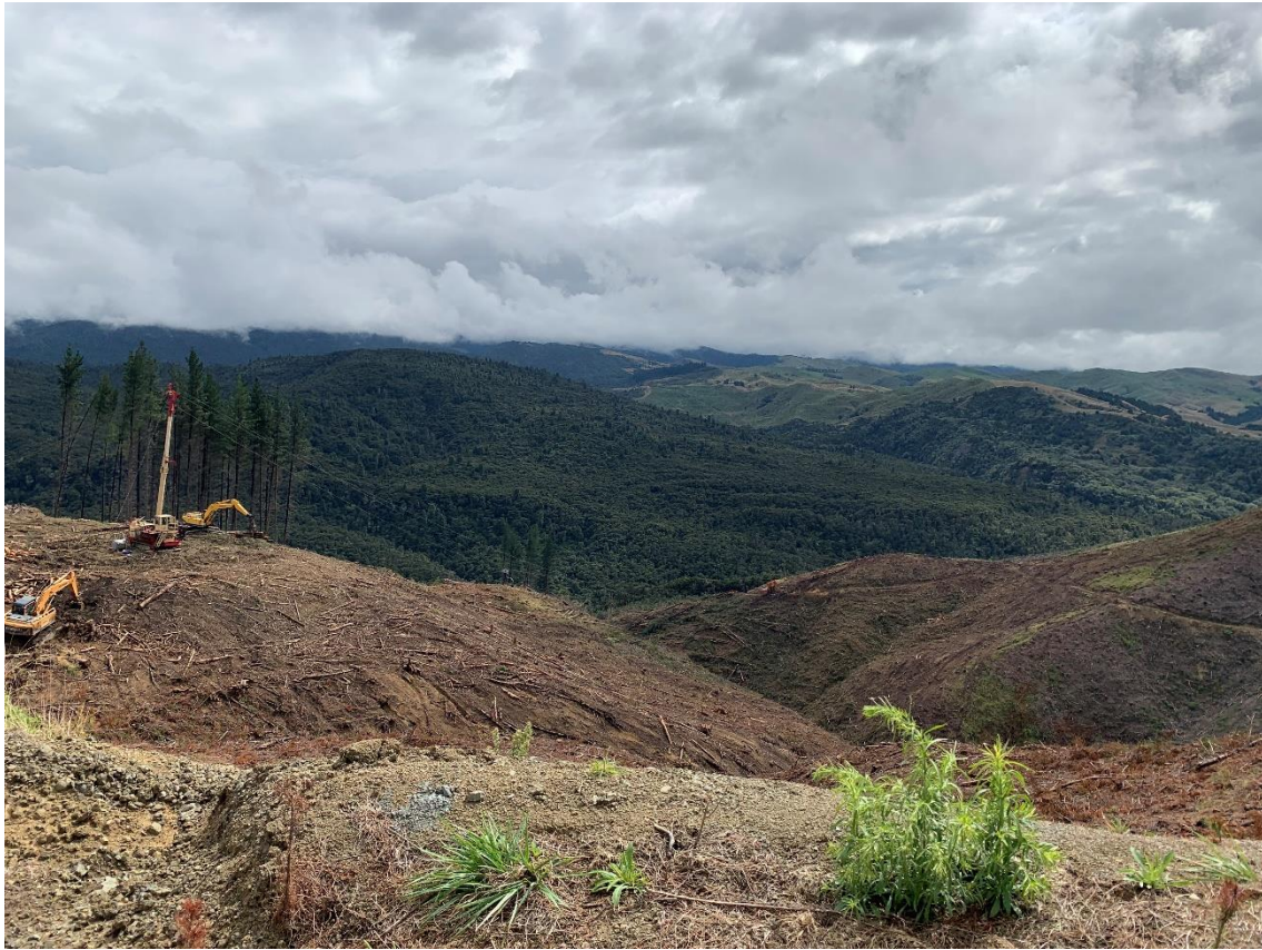
Photo 5: Log 11 hauler pulling Setting 7.
