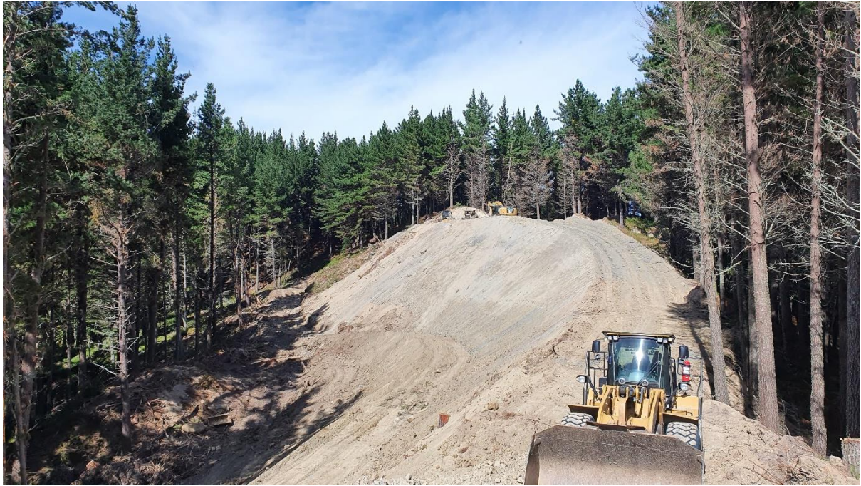
Photo 3: Setting 500, earthworks crew beginning works on Landing 10.
