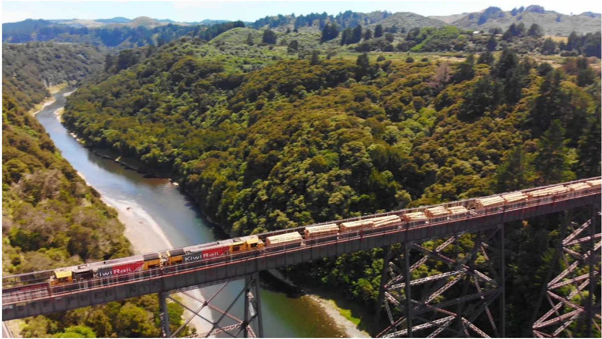
Photo 1: Log train over the Mohaka River on its way to Napier Port.
