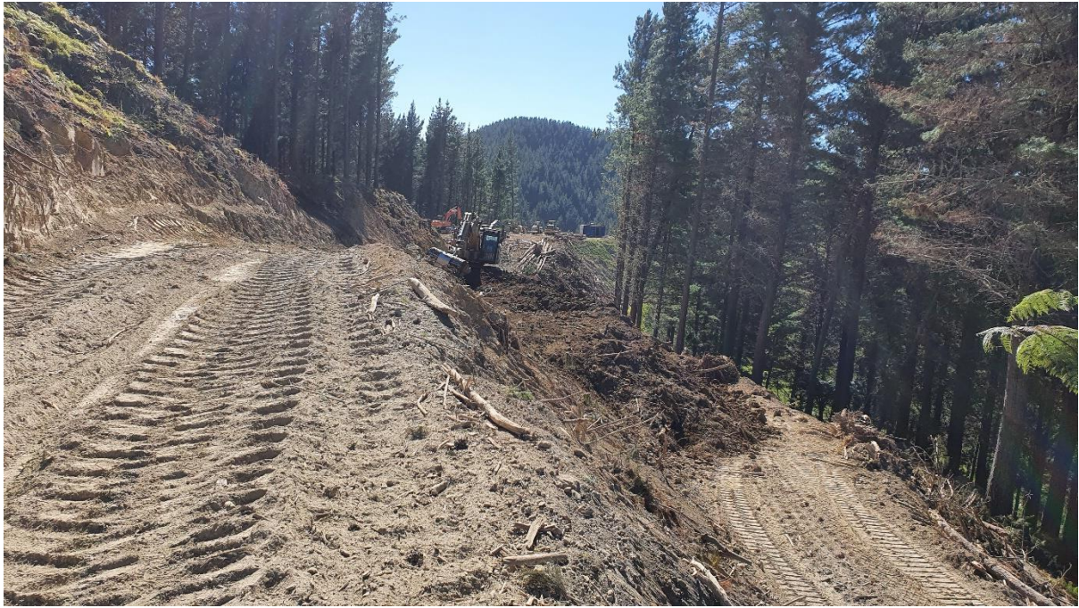
Photo 5: Setting 500, earthworks crew working on formation of Cairns Road.
