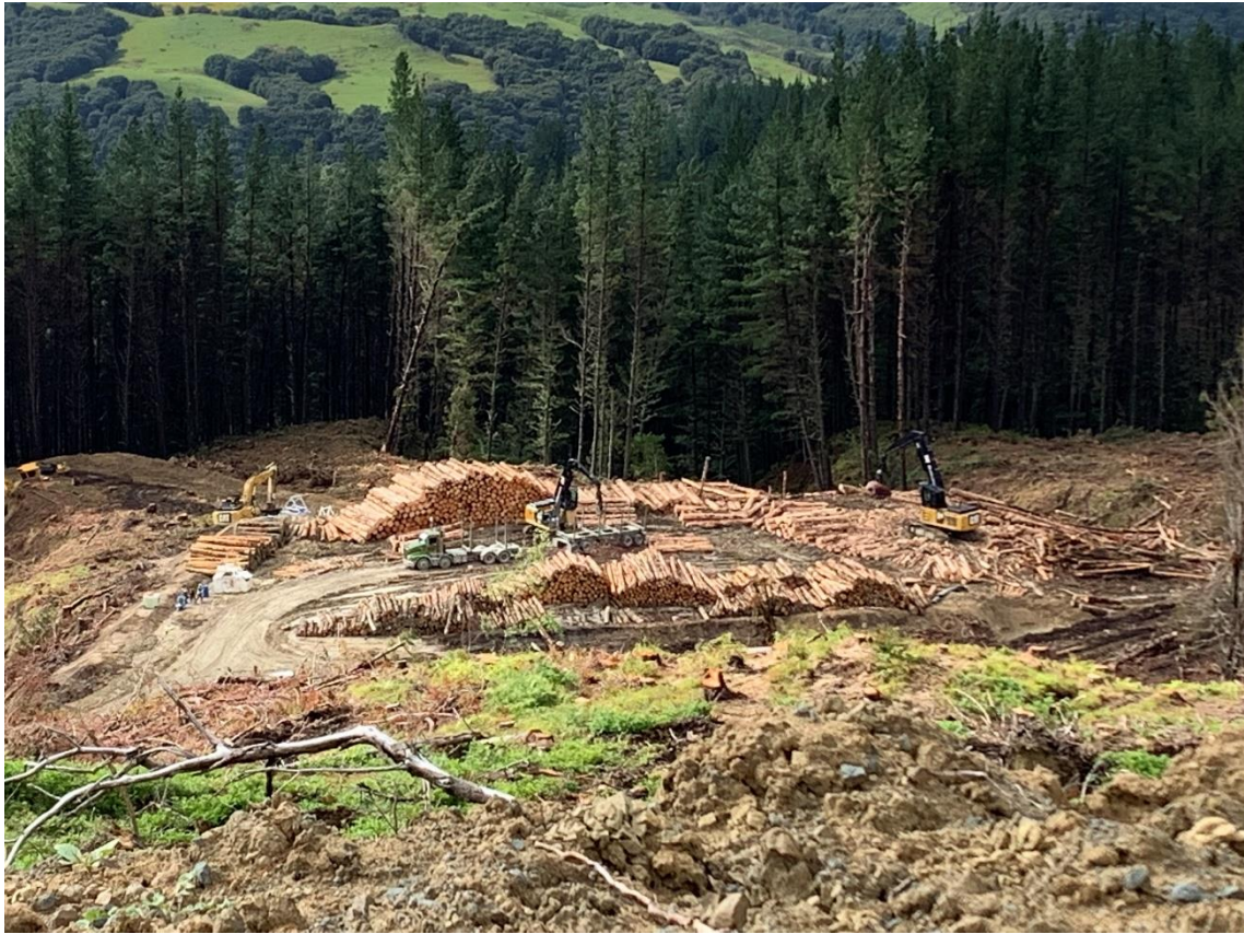
Photo 3: Landing 914 on roadline Setting 505.
