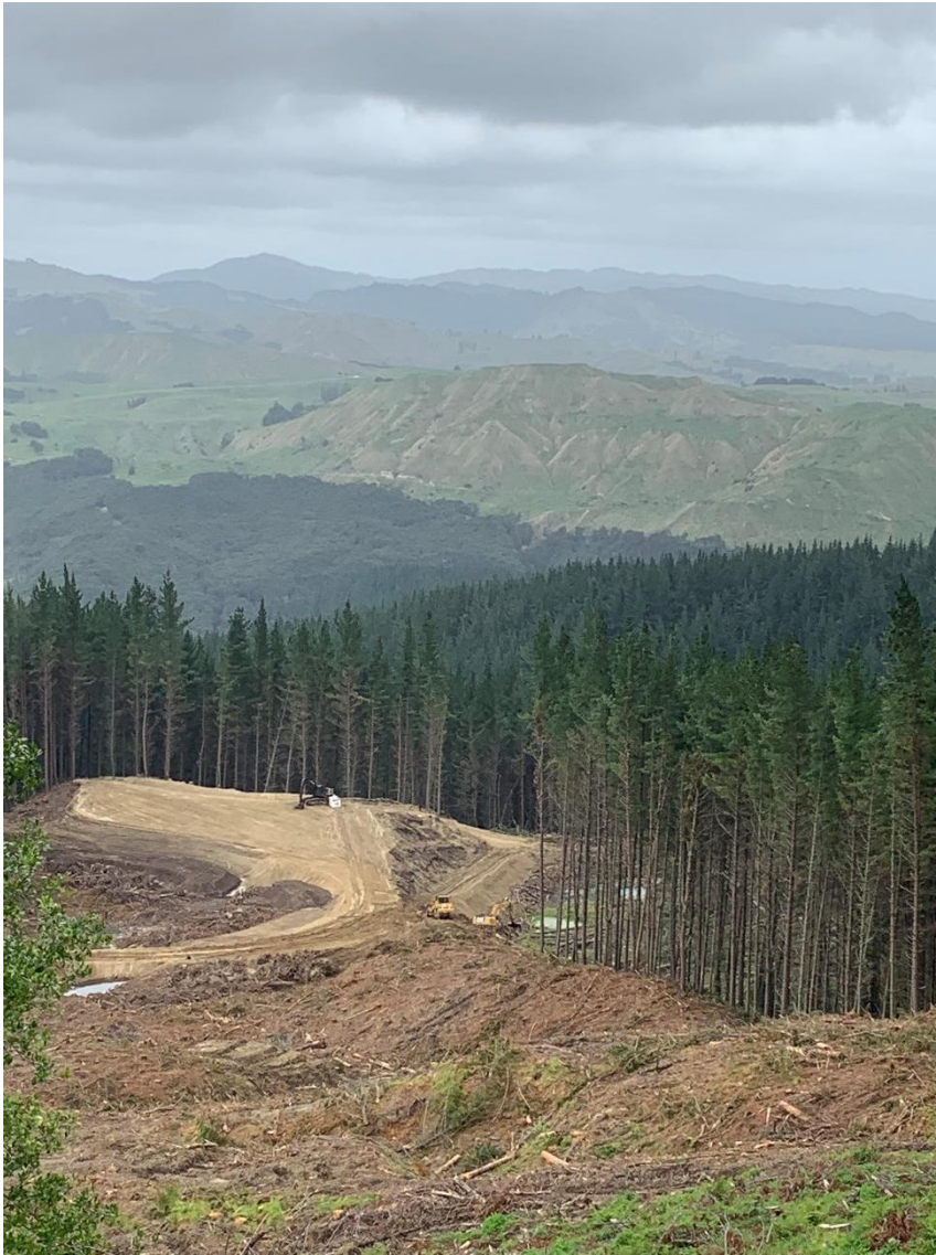
Photo 4: Tahurua Earthmovers working on Landing 915.
