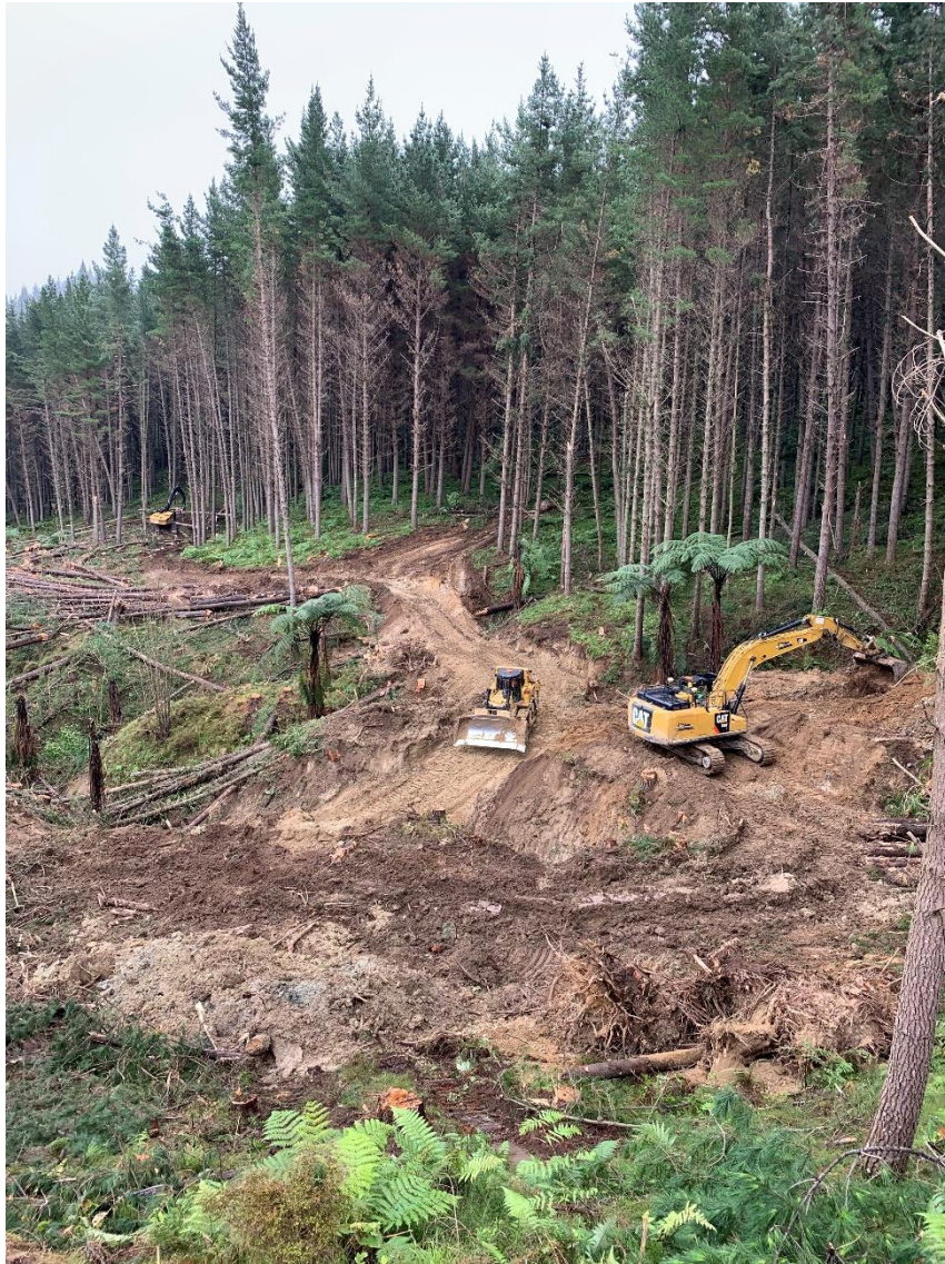
Photo 5: Tahurua Earthmovers working on roadline.
