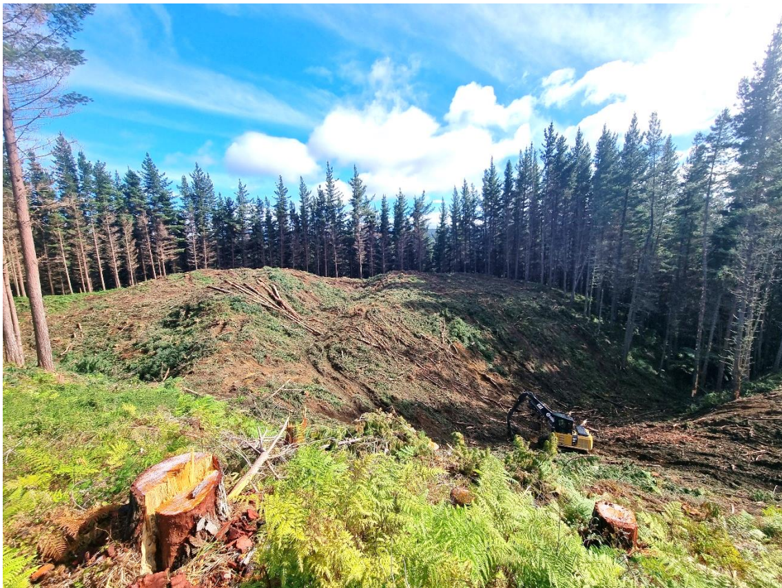
Photo 2: Roadline volume section being cut.
