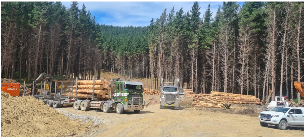
Photo 2: Loading out on Landing 75.
