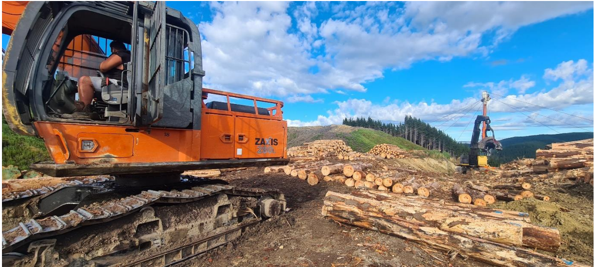
Photo 3: Loadout machine on Landing 4.
