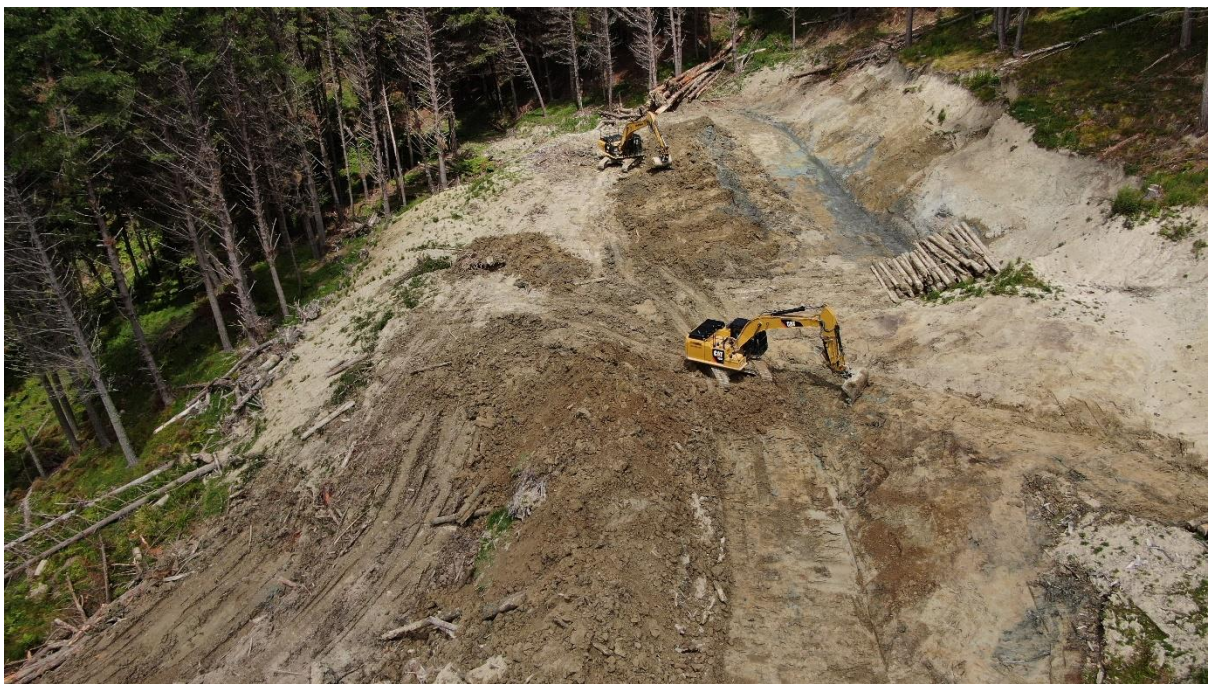
Photo 6: Setting 500, machines preparing Landing 22 for the logging crew to move to next.
