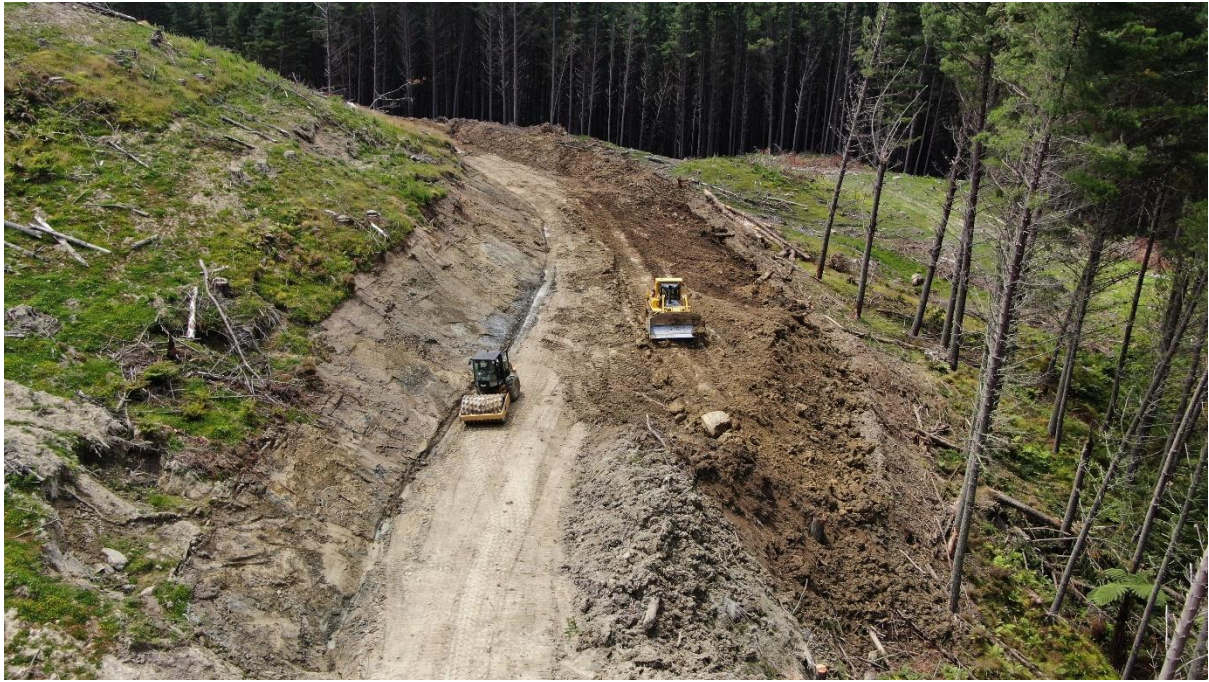
Photo 5: Setting 500, roller and D85 working on section of road to get access between Landings 17 and 22.
