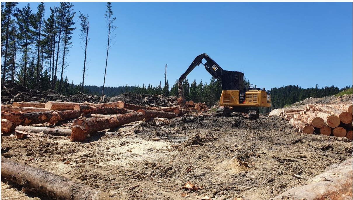
Photo 2: Stacking logs on Landing 17 after manual processing and grading.
