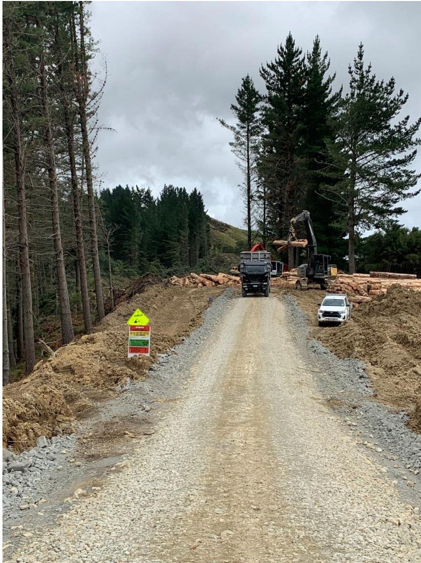
Photo 2: Log 16 working on temporary landing.
