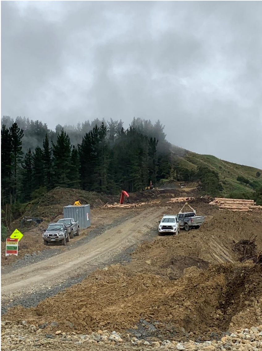
Photo 5: Log 16 operations with earthmovers in the background.
