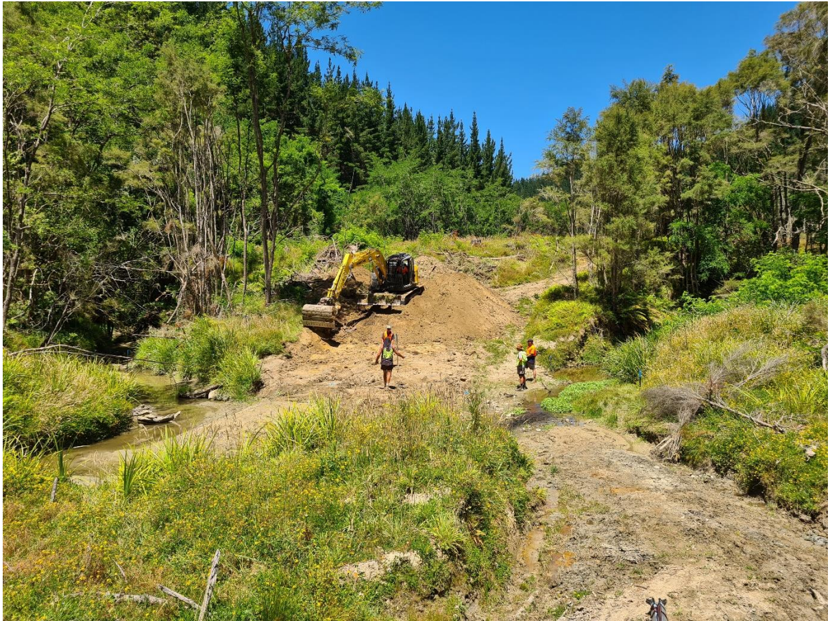
Photo 3: Long Ridge / Ashdown crossing installation.
