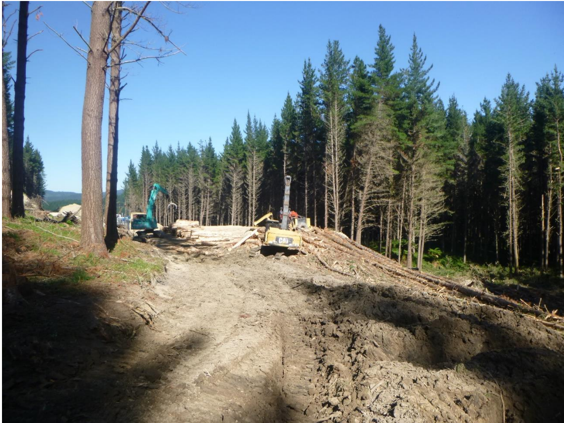
Photo 1: Ngaio Contracting on Landing 4, Setting 500.
