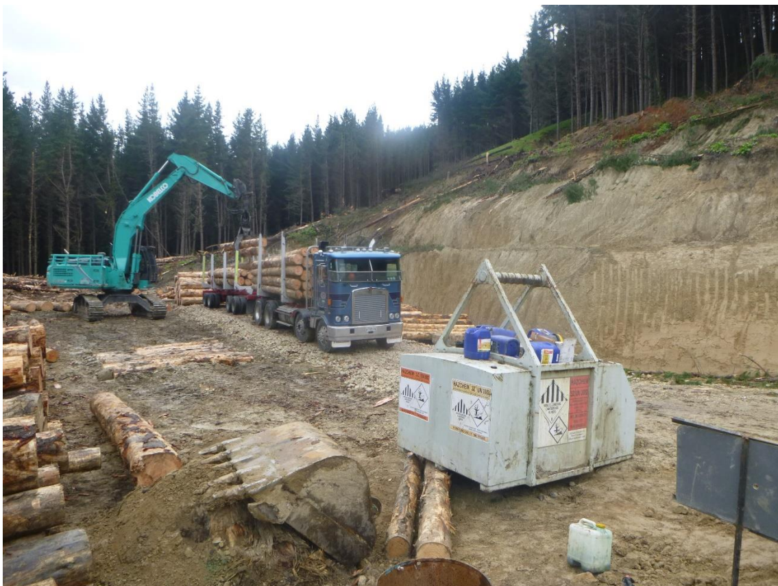
Photo 4: Cutting Setting 500 and loading up on Landing 4.
