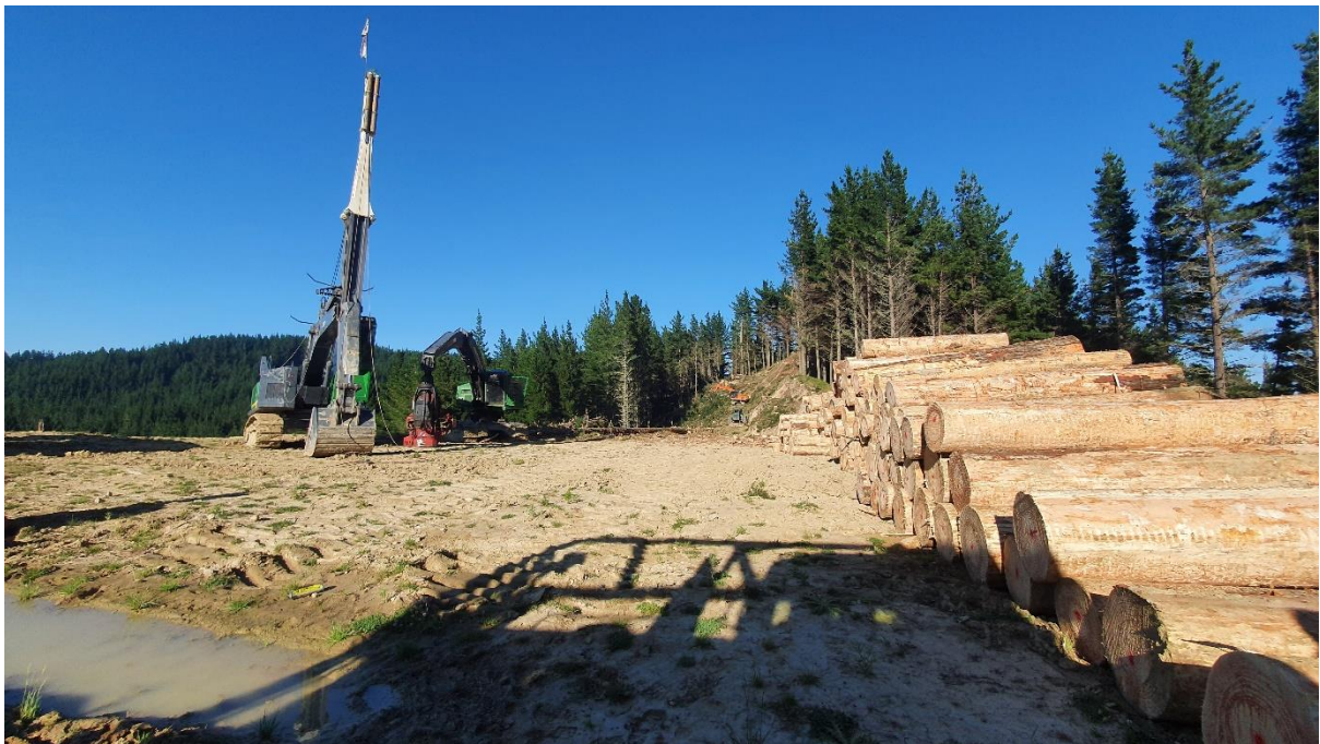
Photo 2: Crew beginning roadline operations from Landing 30 to Landing 10, Setting 500, Cairns Road after the Christmas break.
