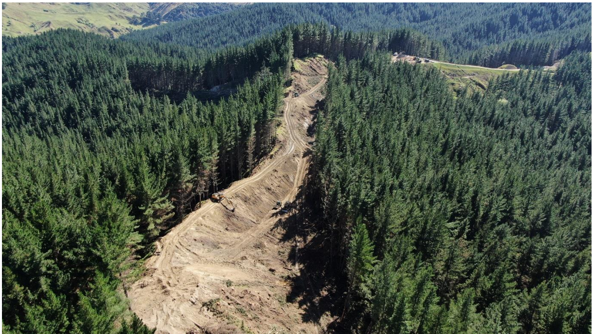
Photo 4: Setting 500, Cairns Road. Earthworks crew beginning works on Landing 10 and looking back towards Landing 30.
