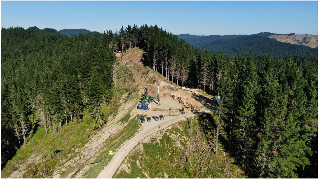
Photo 3: Setting 500, roadlining from Landing 30 through to Landing 10.
