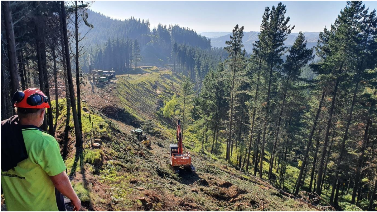
Photo 1: Walking roadline Setting 500 with contractor.
