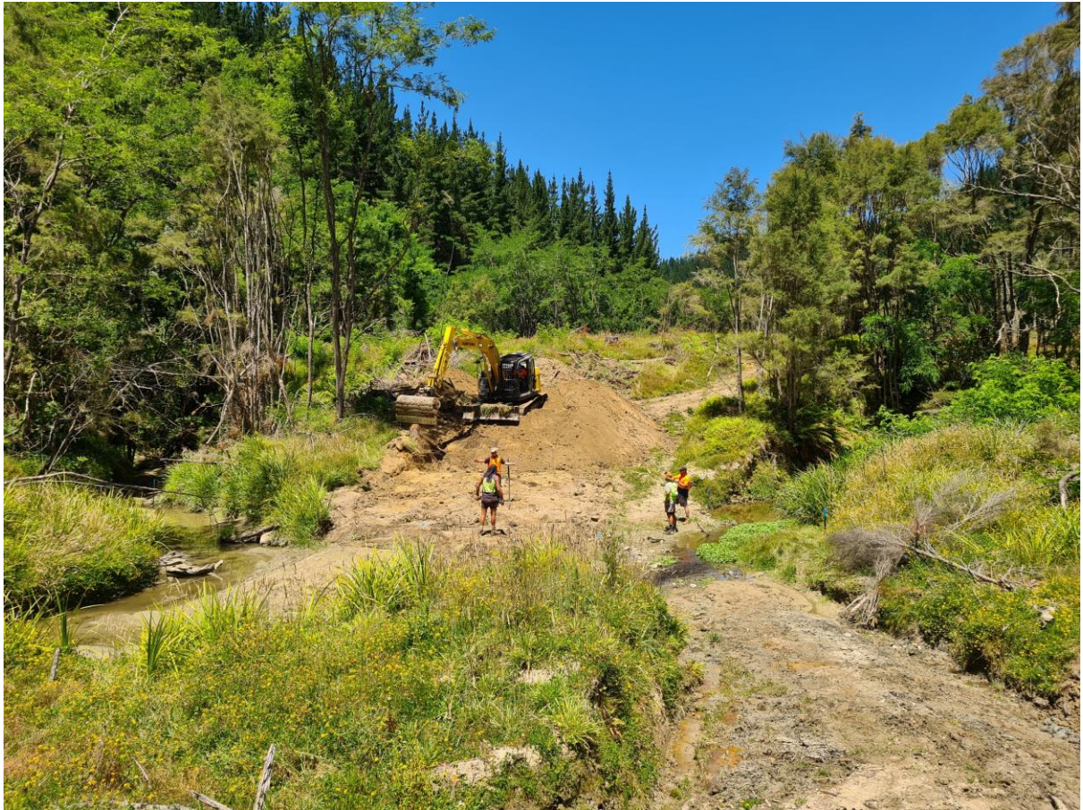
Photo 1: Ashdown / Long Ridge crossing installation.
