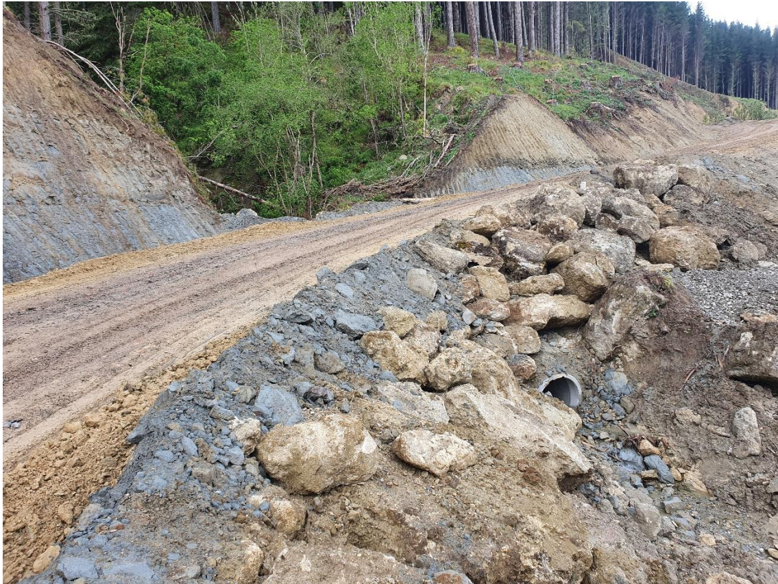
Photo 1: Culvert completion allowing access to Landing 14, Aitken Rd.
