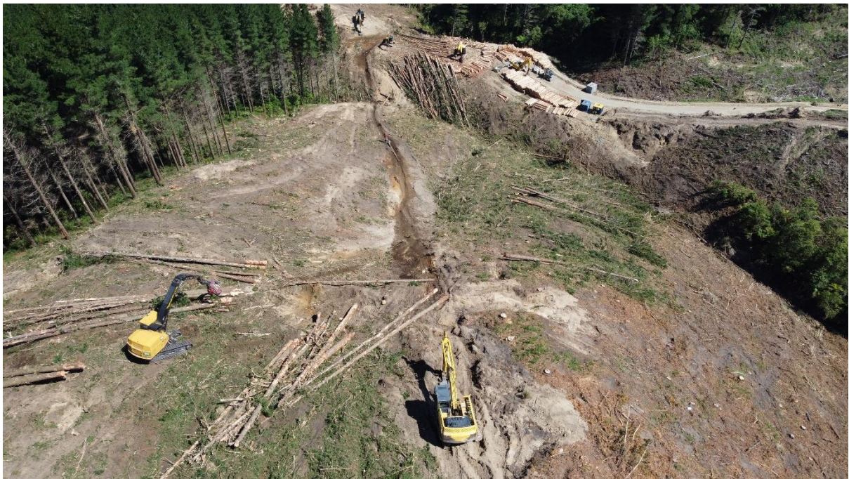
Photo 4: Looking at tail end of operation looking down haul line back towards harvestline.
