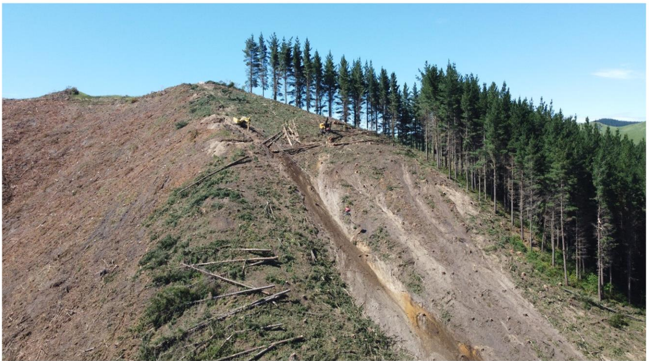
Trees being shovelled under the haul line.
