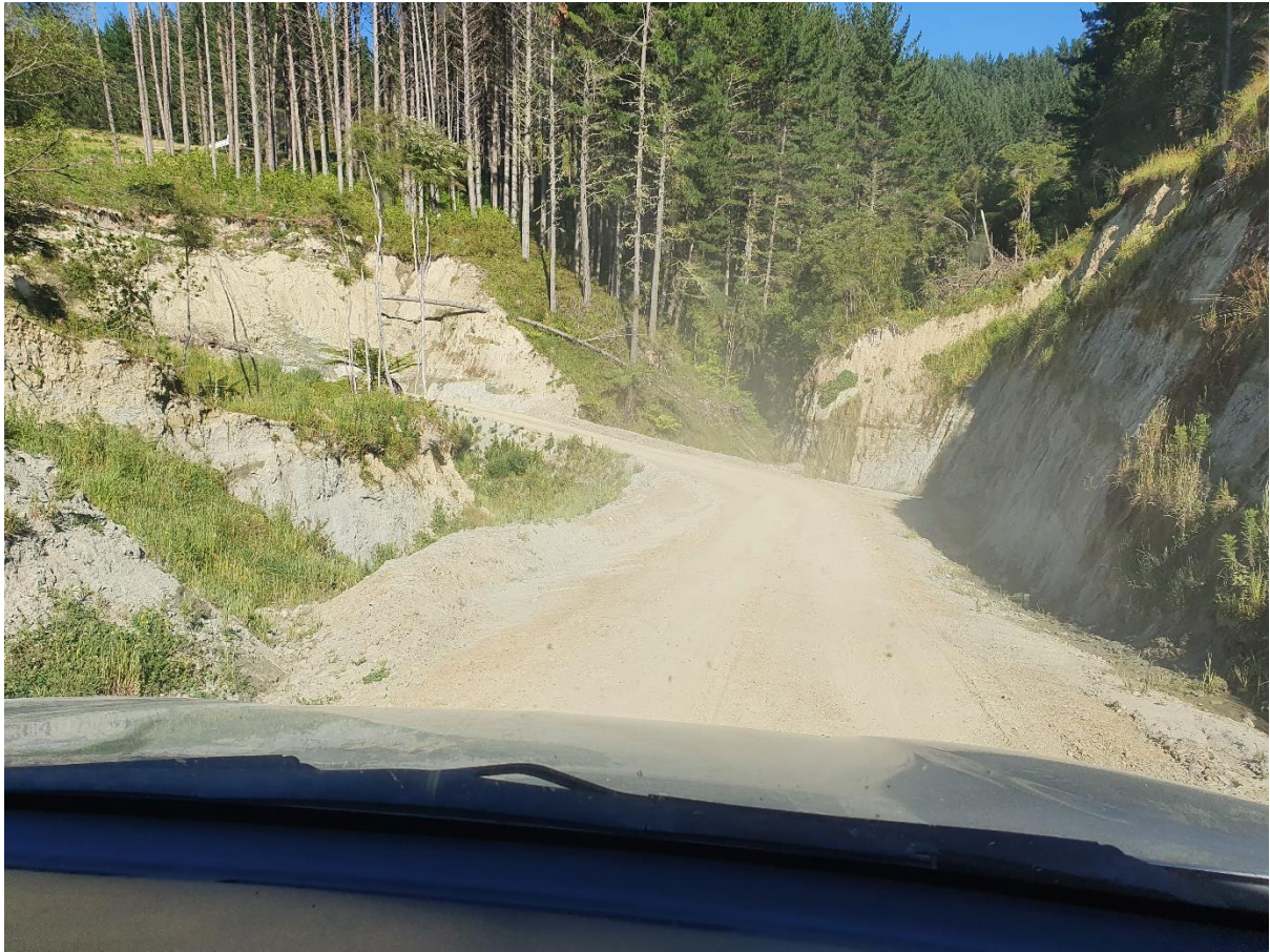
Photo 1: A well-constructed pavement running into the crossing between Landings 7 and 8 in Setting 500.
