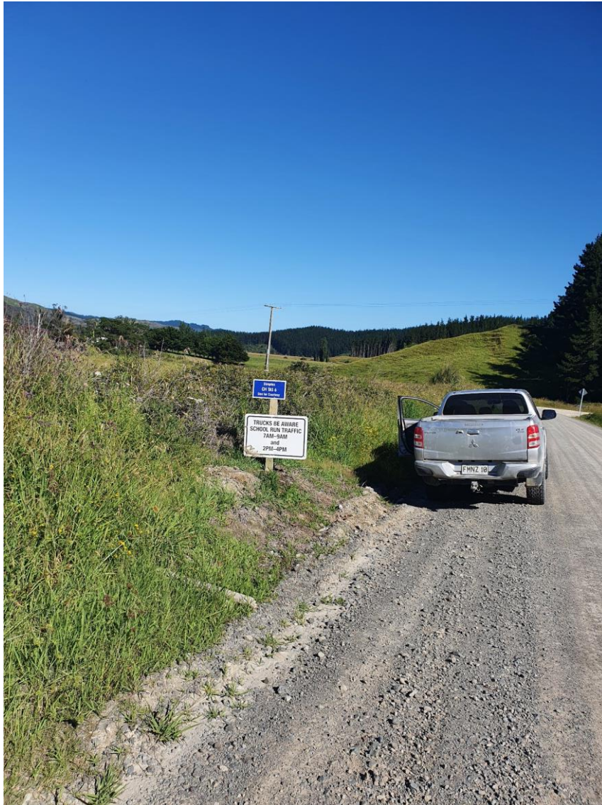
Photo 3: Installing road markers along Waihua Valley Road to increase the safety of our forest traffic and local traffic.
