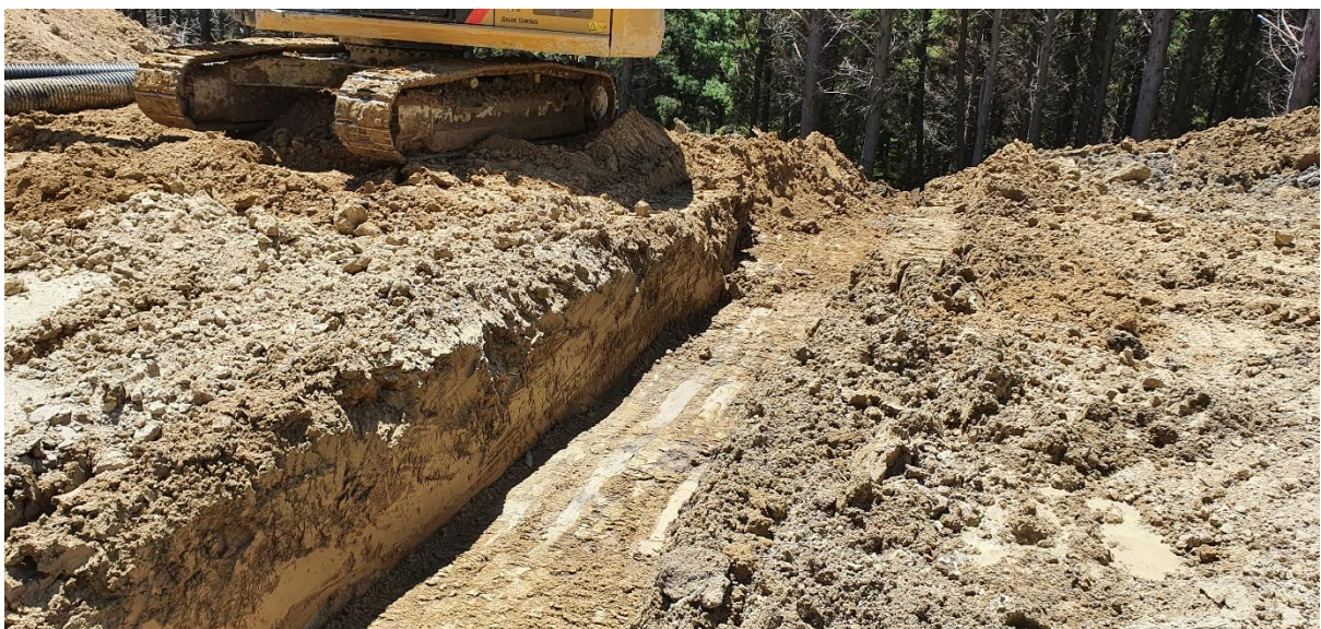
Photo 4: Undertaking culvert installation between Landings 17 and 22 on Murray Road, Setting 500.
