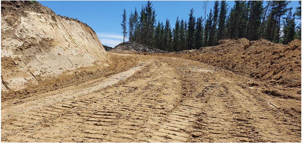
Photo 5: Undertaking pavement formation between Landings 17 and 22 on Murray Road, Setting 500.
