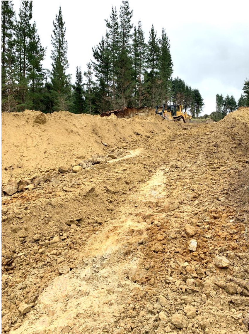
Photo 2: Tahurua Earthmovers building Landing 107.
