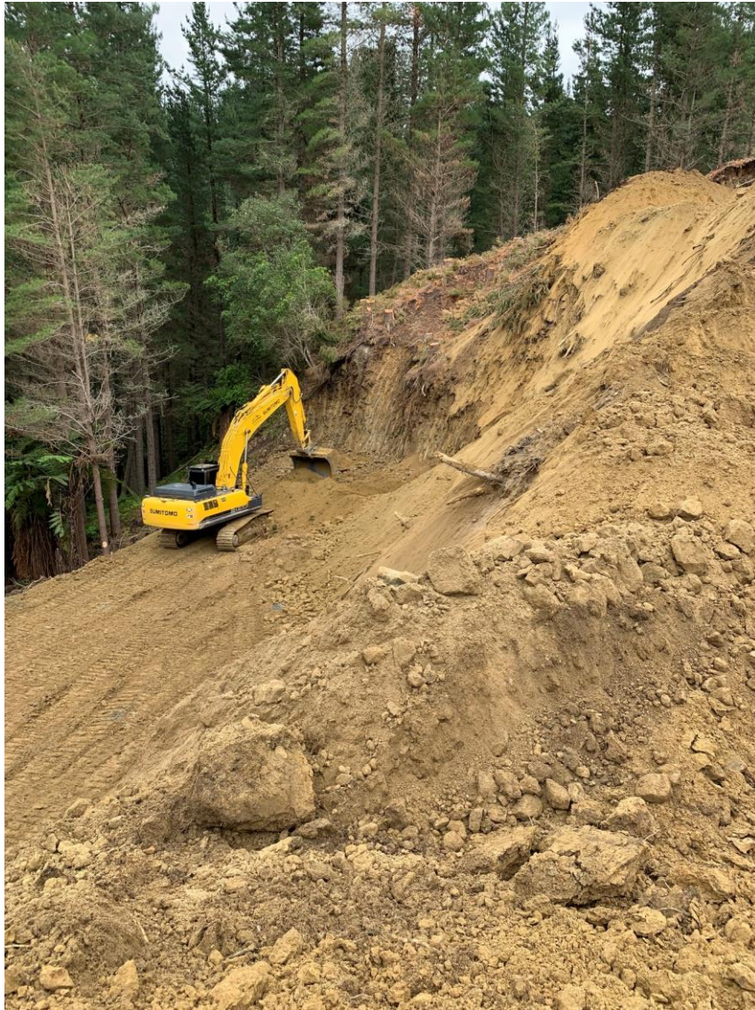
Photo 3: Tahurua Earthmovers building Landing 107.
