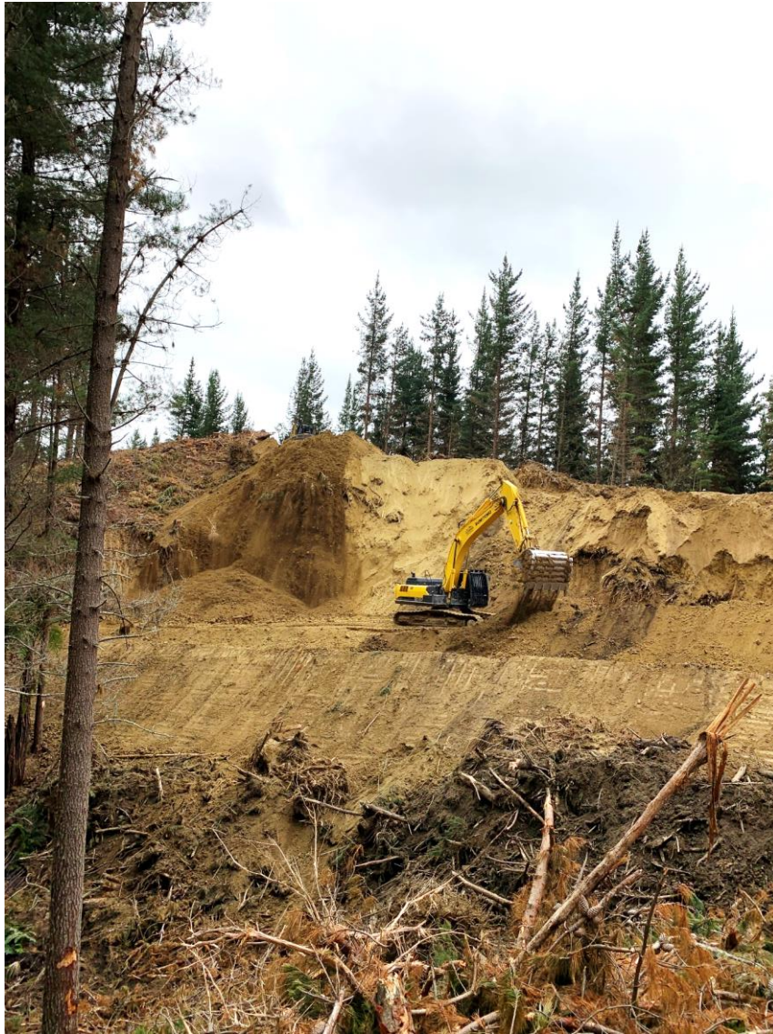
Photo 4: Tahurua Earthmovers building Landing 107.
