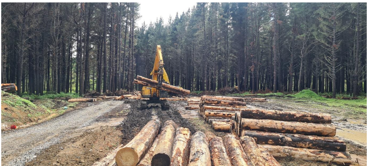
Photo 6: Stacking wood on Landing 34.
