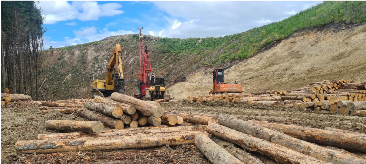
Photo 4: Swing yarder on Landing 21.
