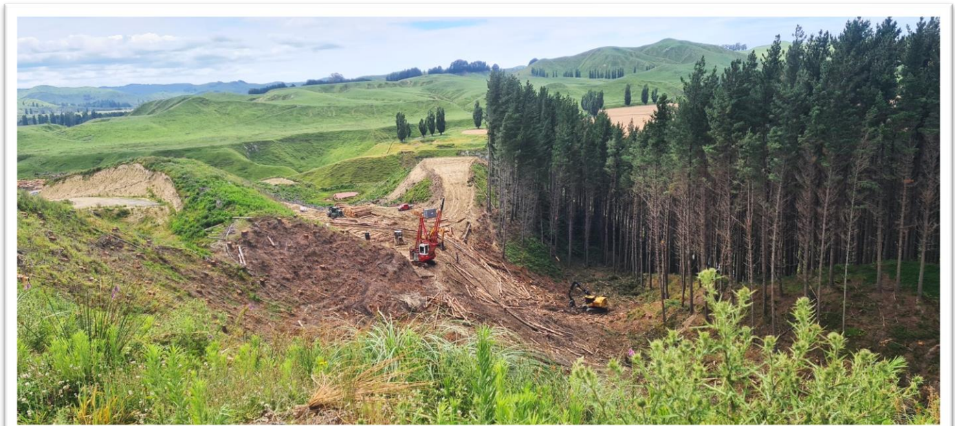
Aerial view of Setting 21.
