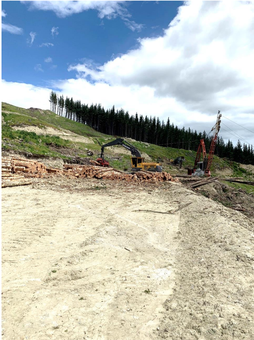
Photo 1: Operations on Landing 205.
