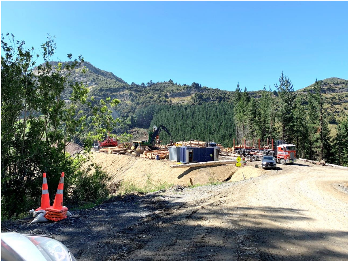
Photo 2: Landing 69, hauler pad operation, trucks being loaded.
