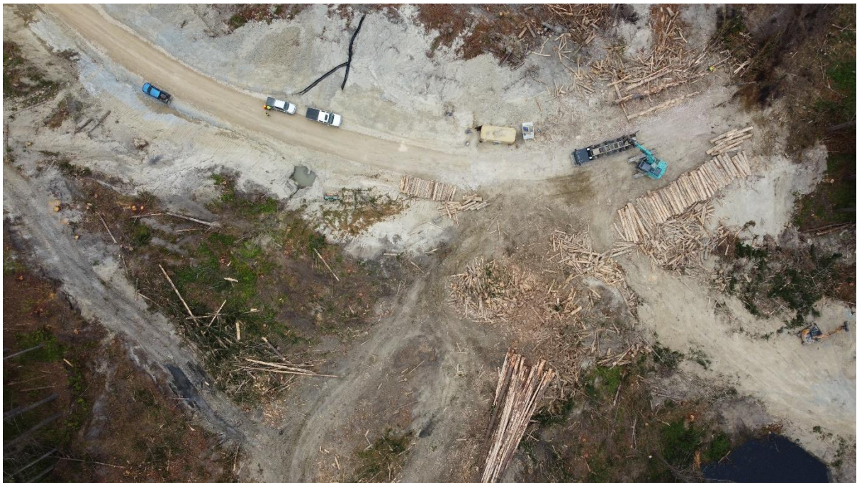
Photo 2: Aerial view of temporary landing above bridge site.
