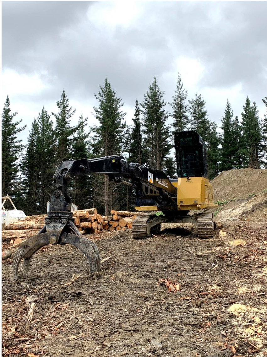
Photo 2: CAT loader on Landing 913.
