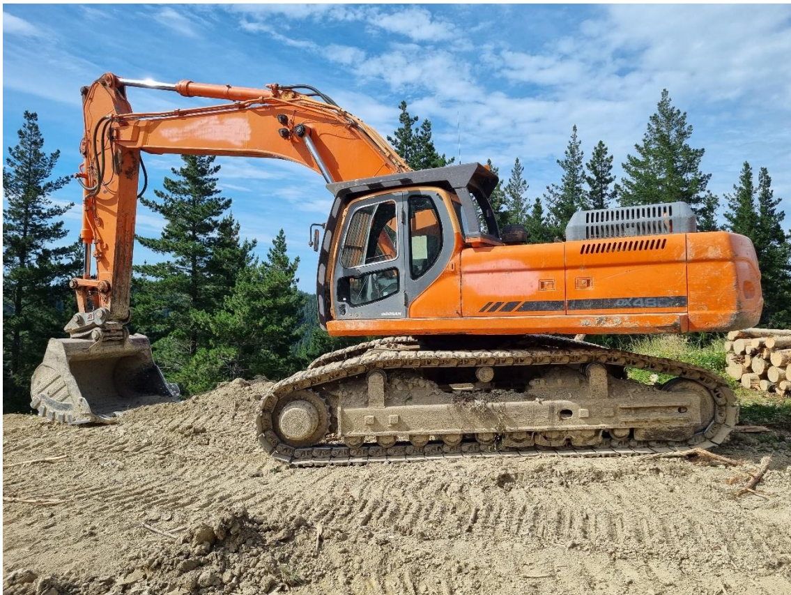
Photo 4: Large excavator used for moving large hills sides to push tracks in quickly for two-staging tracks.
