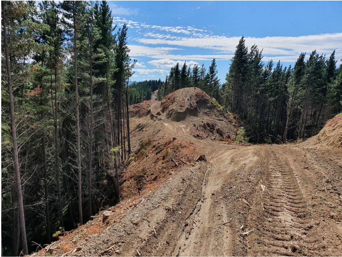
Photo 7: Ridge top roadline felled ready for road formation team to come in and build a road.
