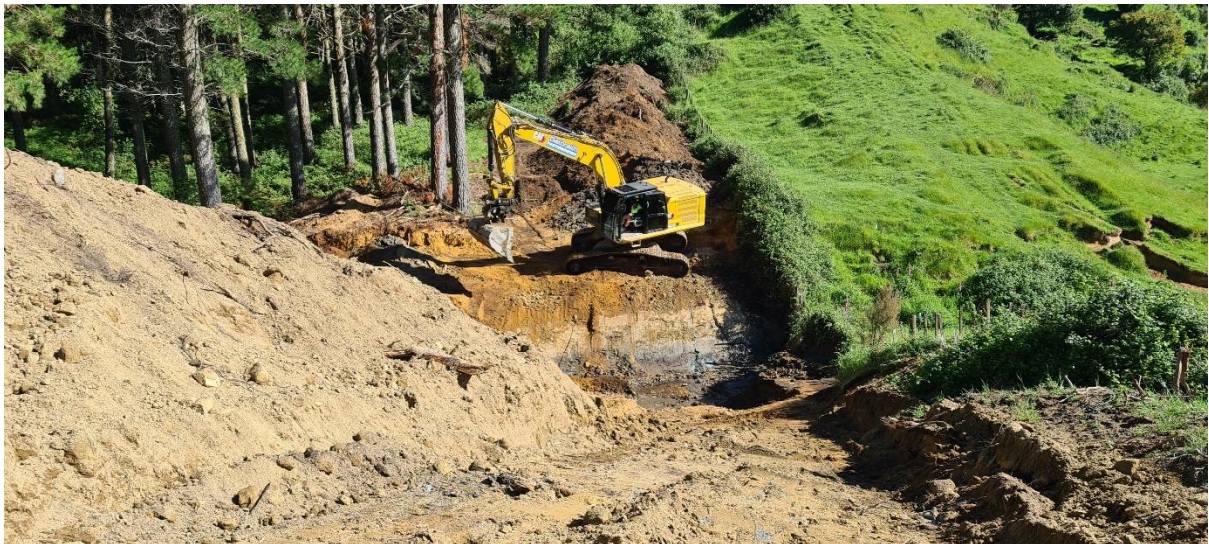
Photo 2: Installation of culvert above Landing 25.
