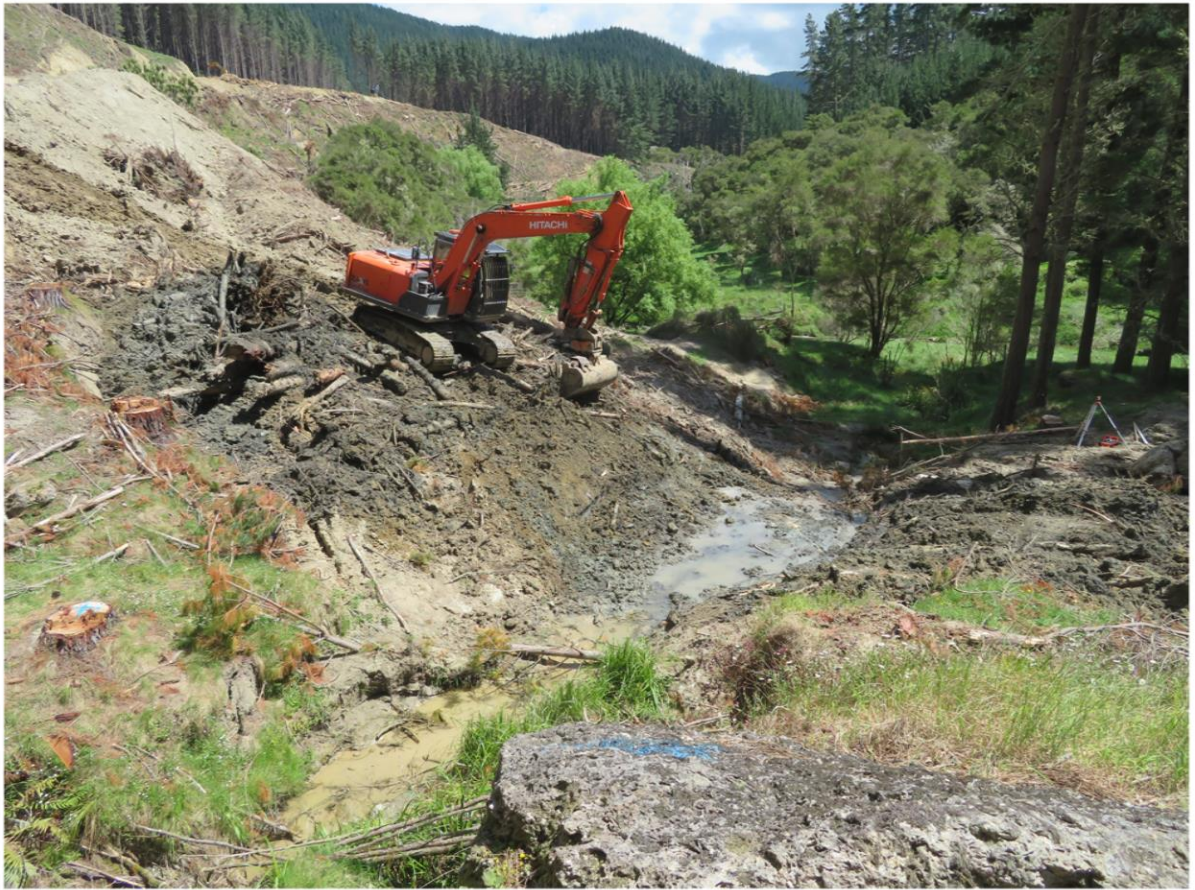
Crossing installation between Landings 13 and 14 on Aitken Road.
