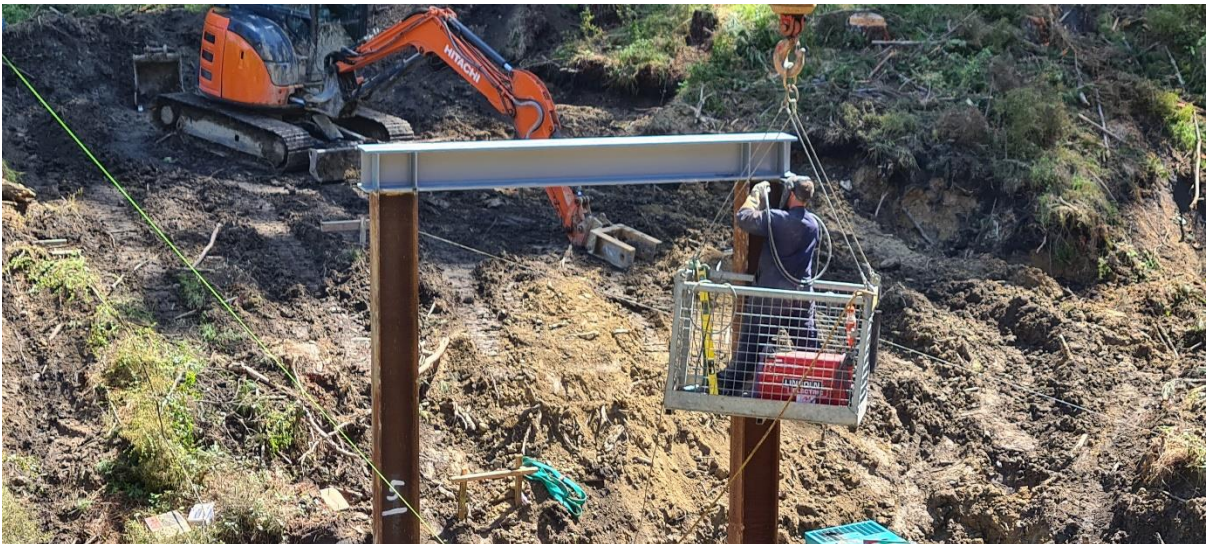
Photo 2: Crossbars being welded on bridge piles.
