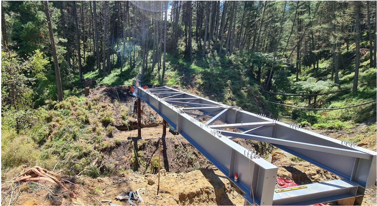
Photo 3: Bridge placed on piles.
