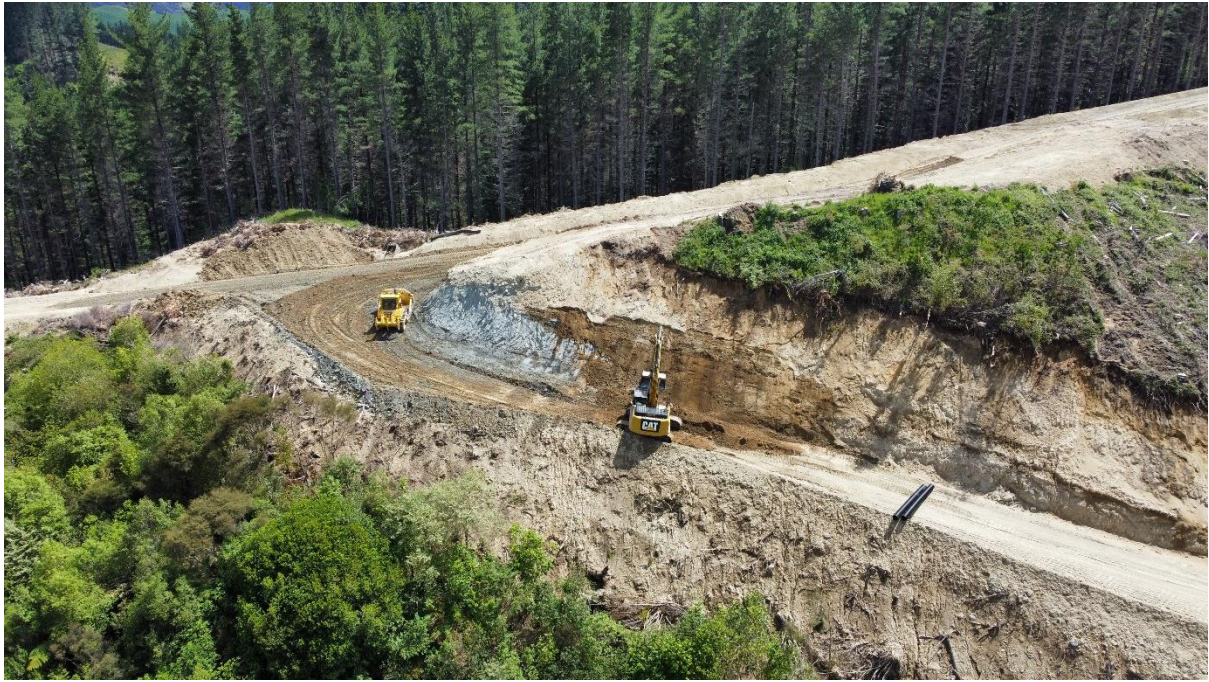
Photo 1: Snowdon Road being formed.
