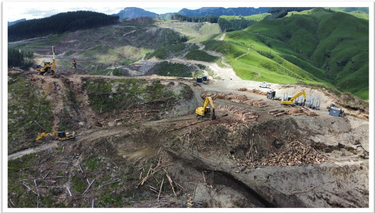
Operations on Landing 150.
