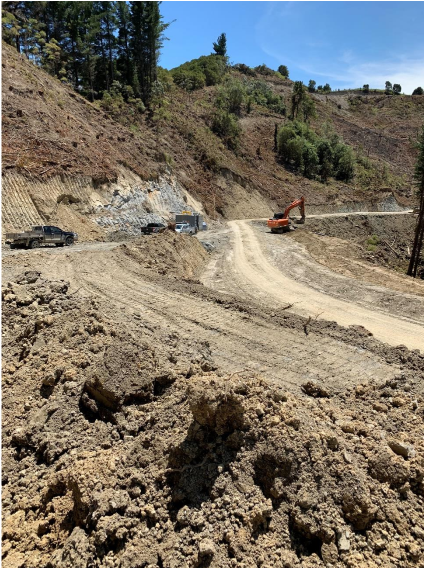
Photo 3: Construction of the junction at McCoy and Richardson Roads.
