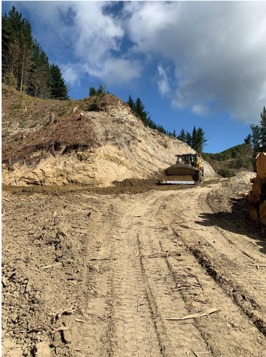
Photo 2: Construction of Richardson Road.
