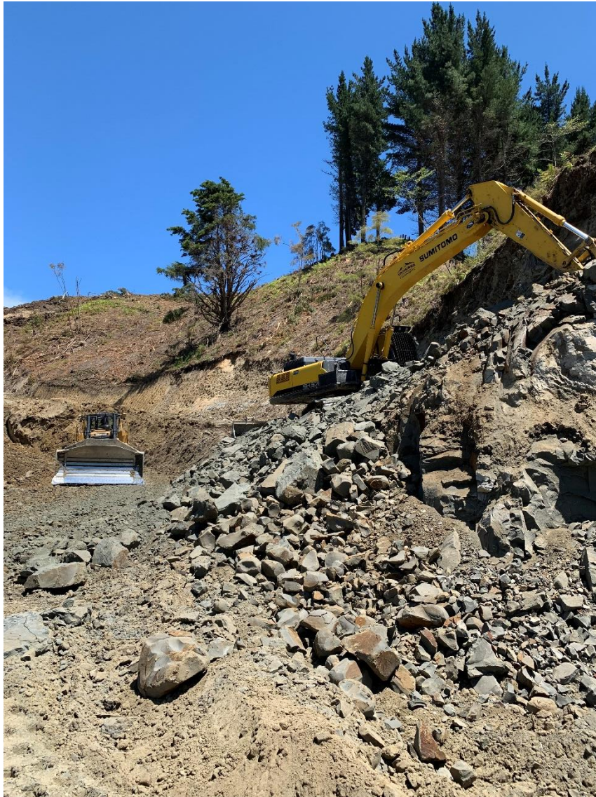
Photo 5: Digging out papa rock, construction of McCoy Road.
