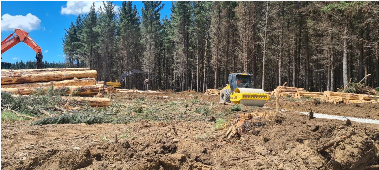
Photo 1: Rolling end of Tutaekuri Road near temporary landing.
