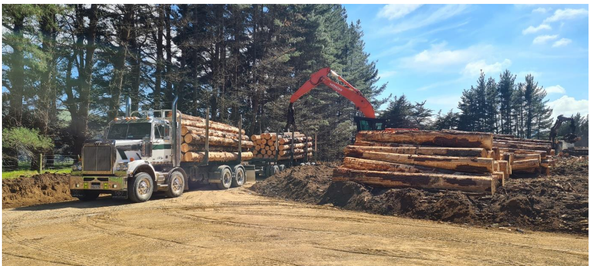
Photo 6: Loading out on temporary Landing 41.
