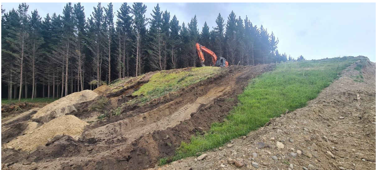
Photo 3: Construction of Landing 34.
