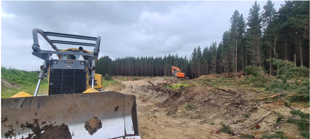
Photo 4: Formation of Tutaekuri Road near temporary Landing 41.
