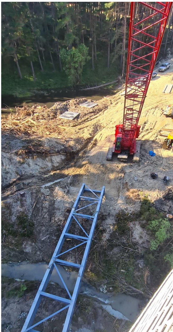
Photo 4: Looking down on the bridge site from the crane cage.
