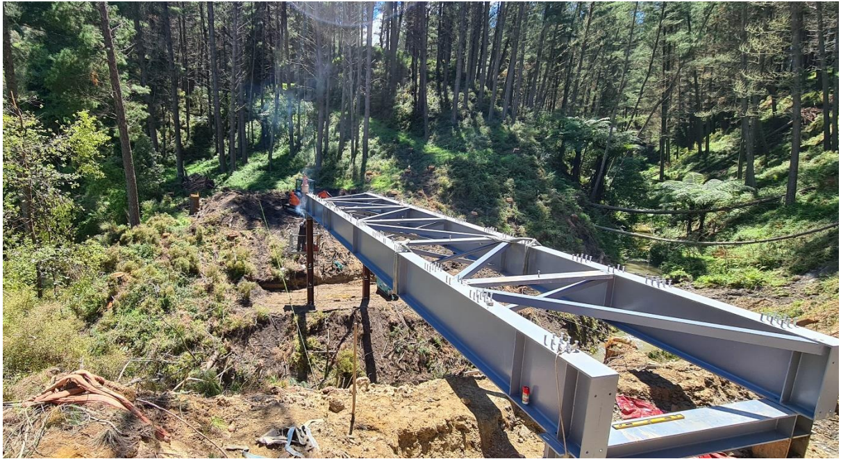
Photo 3: Bridge placed on piles.
