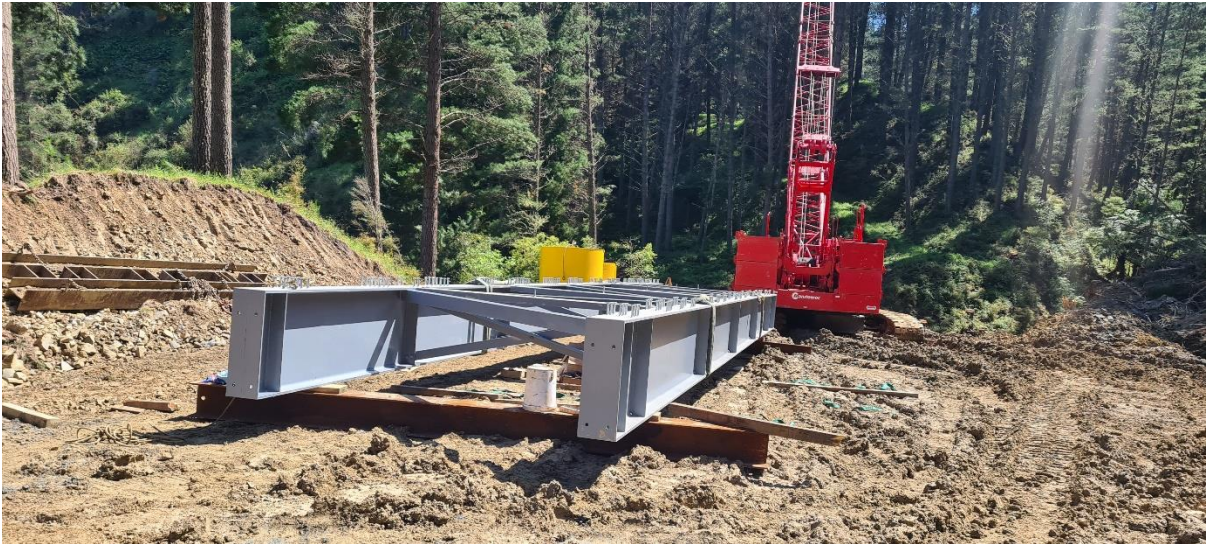
Photo 1: Bridge awaiting installation.
