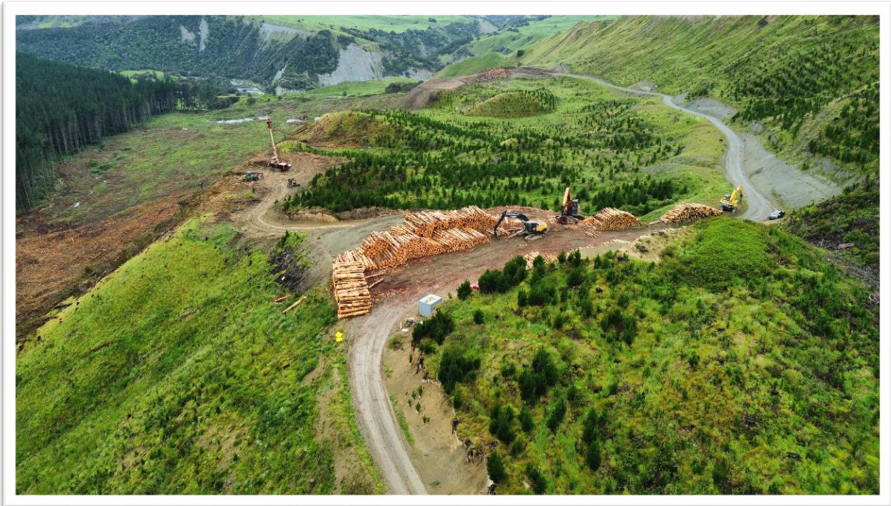
Hauler on Landing 24A and wood stacks on Landing 24.
