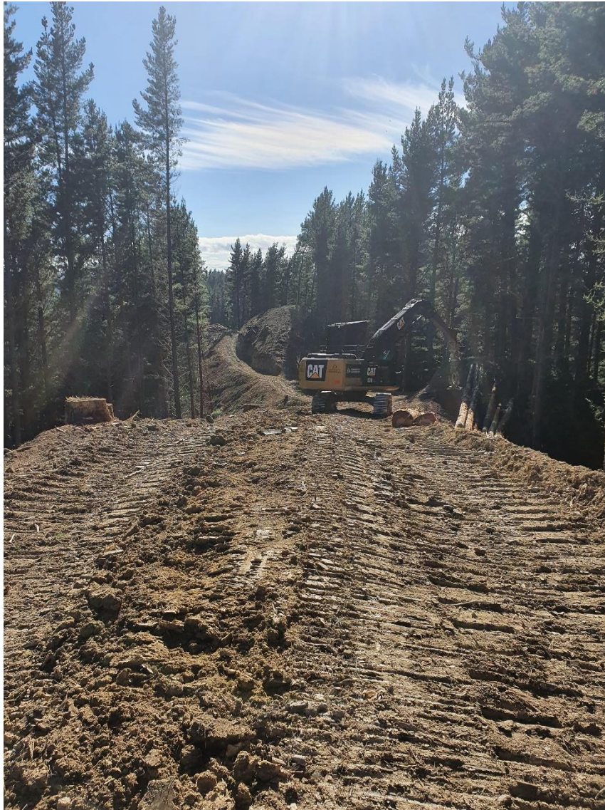
Photo 3: Benching on Douglas Road.
