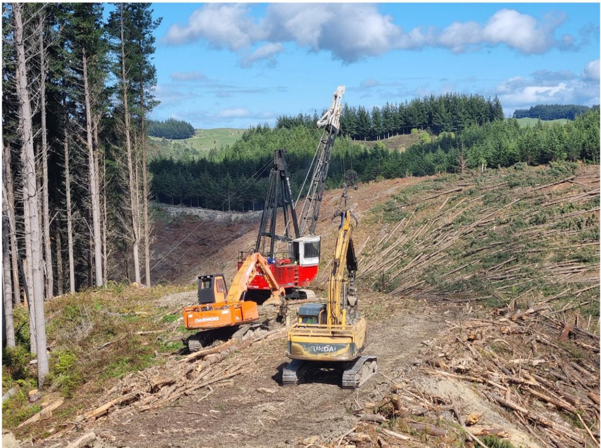
Swing yarder and excavators on Pad 28B retrieving felled stems.
