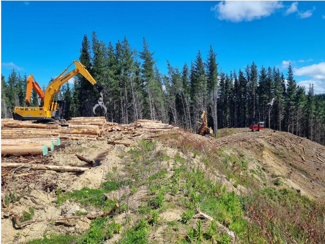
Photo 1: Two-stage operation from Pad 28B to Landing 28.
