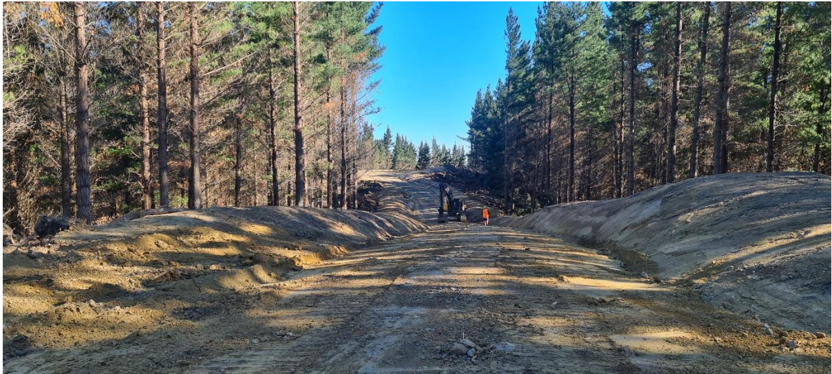
Photo 4: Construction of Magog Road between Landings 87 and 81.
