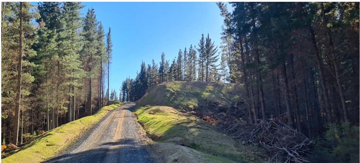
Photo 5: Good result of hydroseeding on Magog Road.
