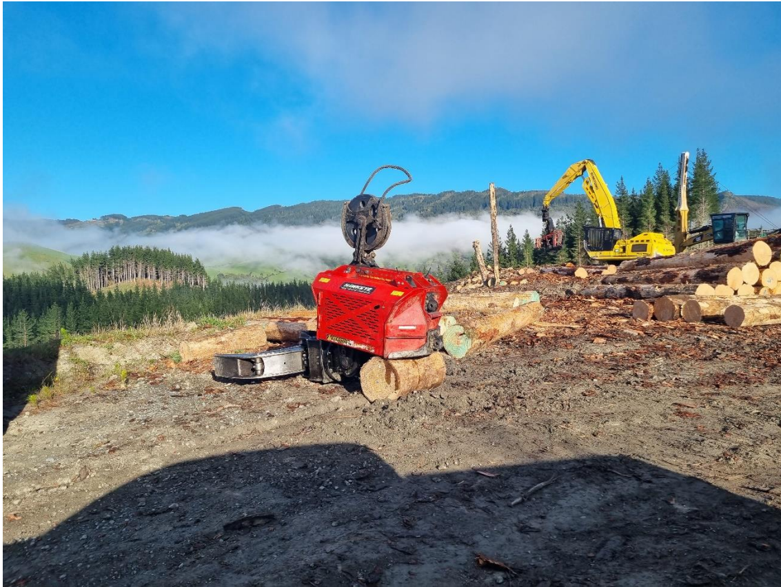
Photo 1: Red mechanised carriage back in action after repairs, this mechanised system enables production to be quicker compared to manual breaking out.
