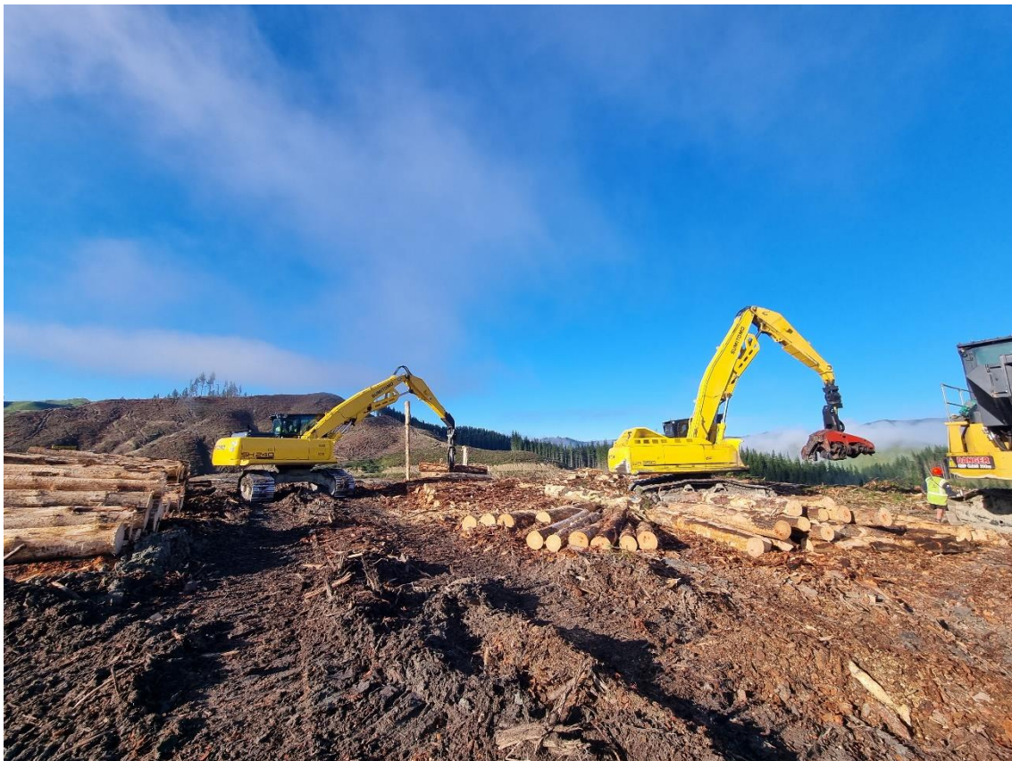
Photo 2: Machines at work on Landing 134.
