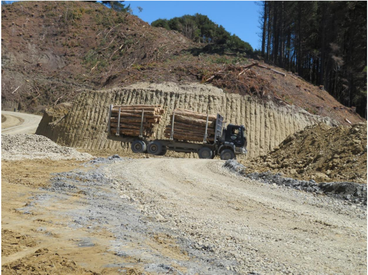
Photo 1: Staging truck going past Landing 103.
