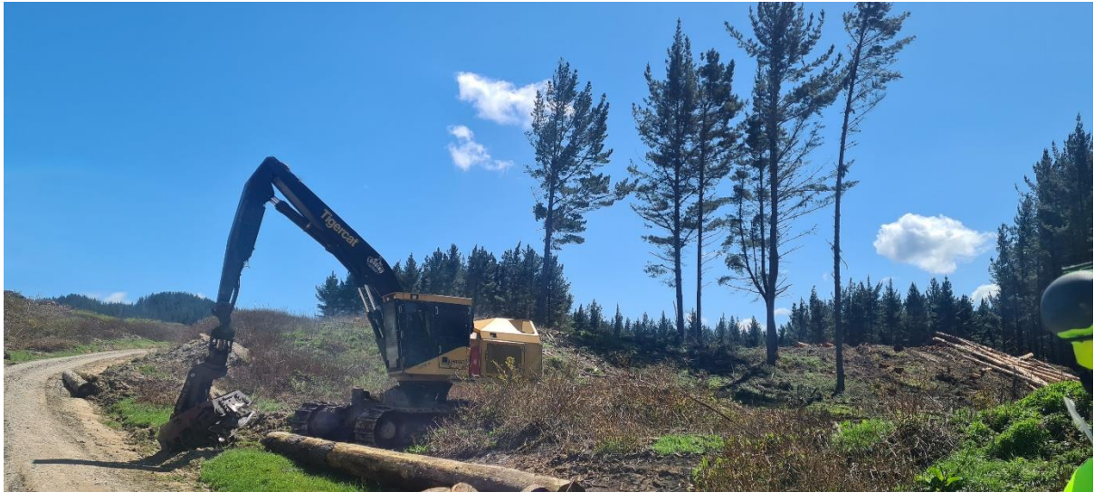
Photo 1: Felling machine sitting above Landing 33.
