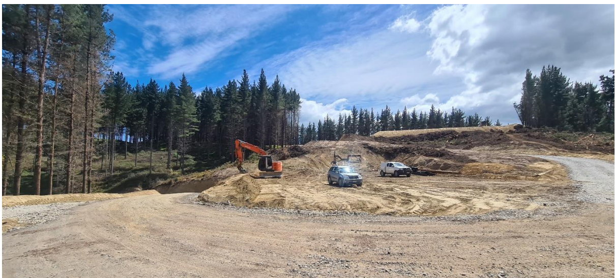
Photo 3: Minor earthworks on Landing 31.
