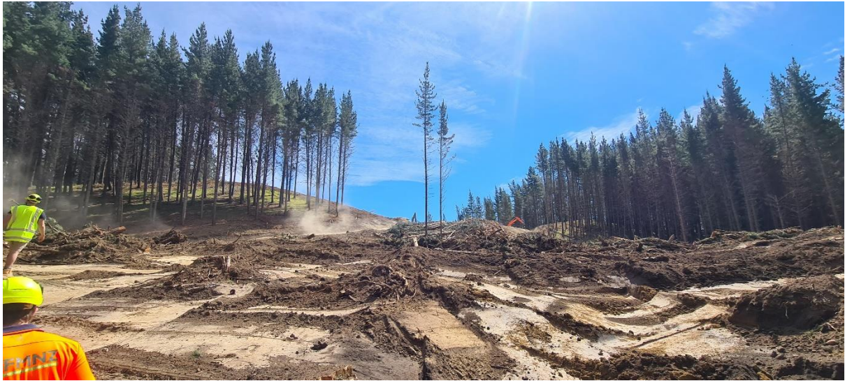
Photo 4: Roadline corridor being cut to Landing 32.
