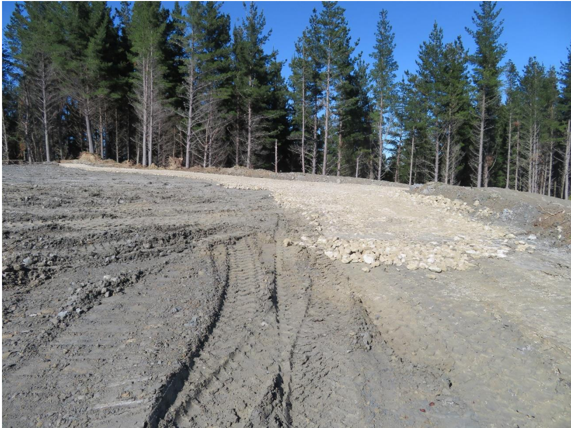
Photo 1: Landing 19 loadout bay.
