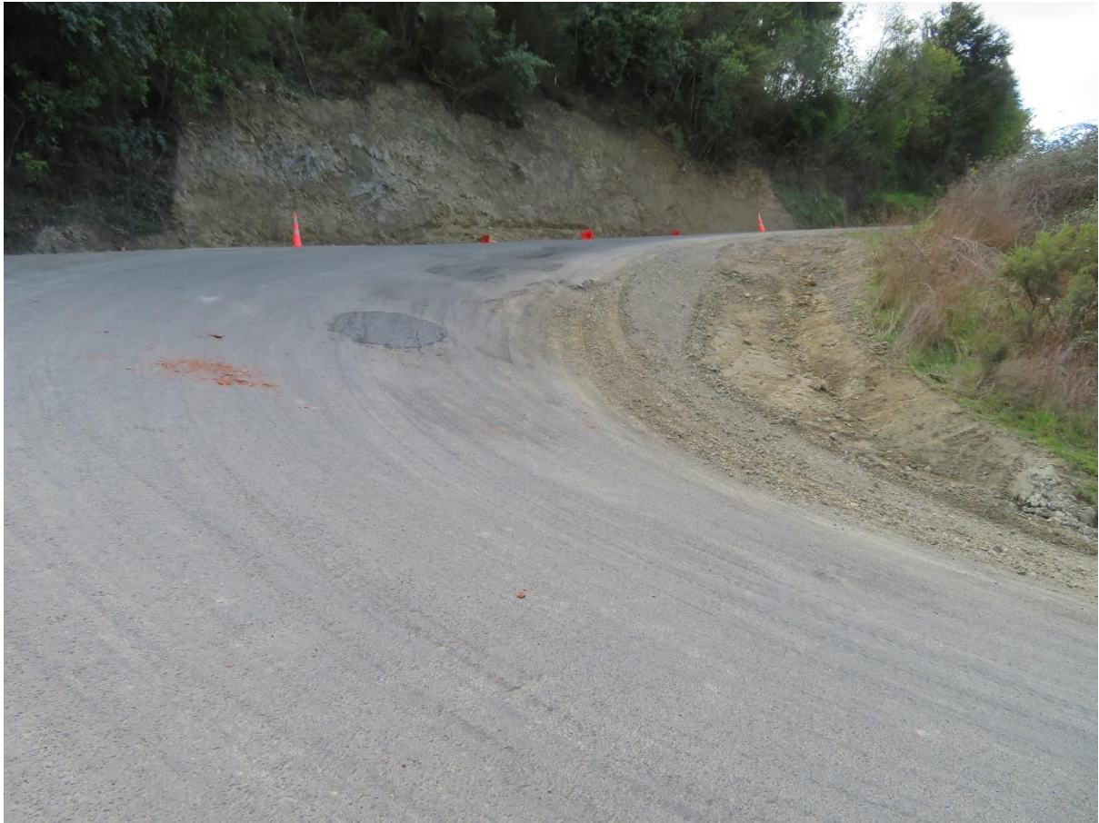
Photo 5: Waireka Road staircase switchback improvements by Wairoa District Council.
