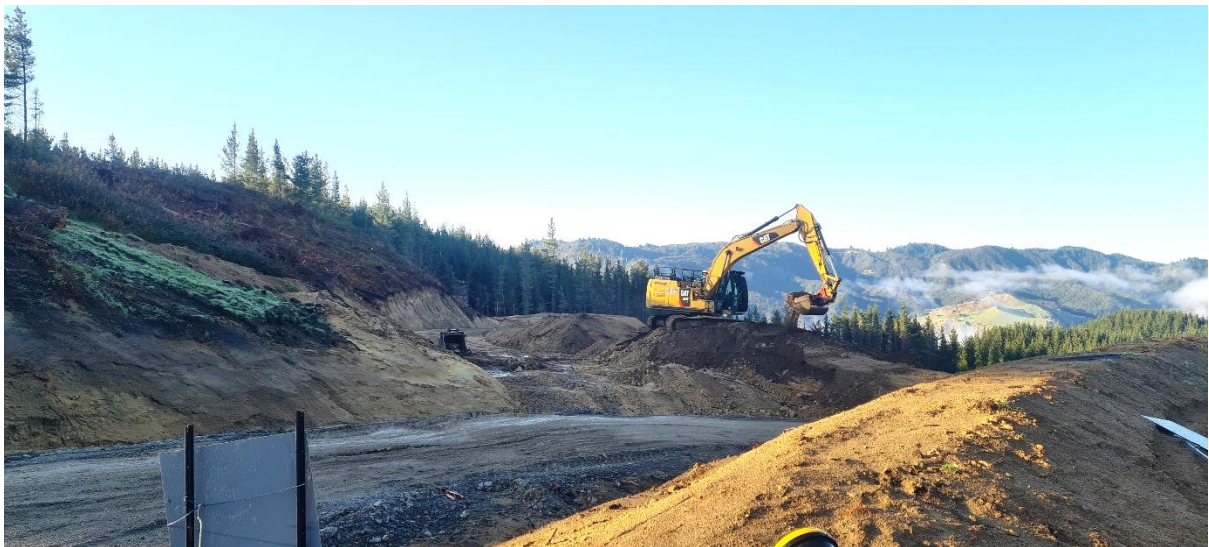
Photo 6: Construction of road to Landing 7.
