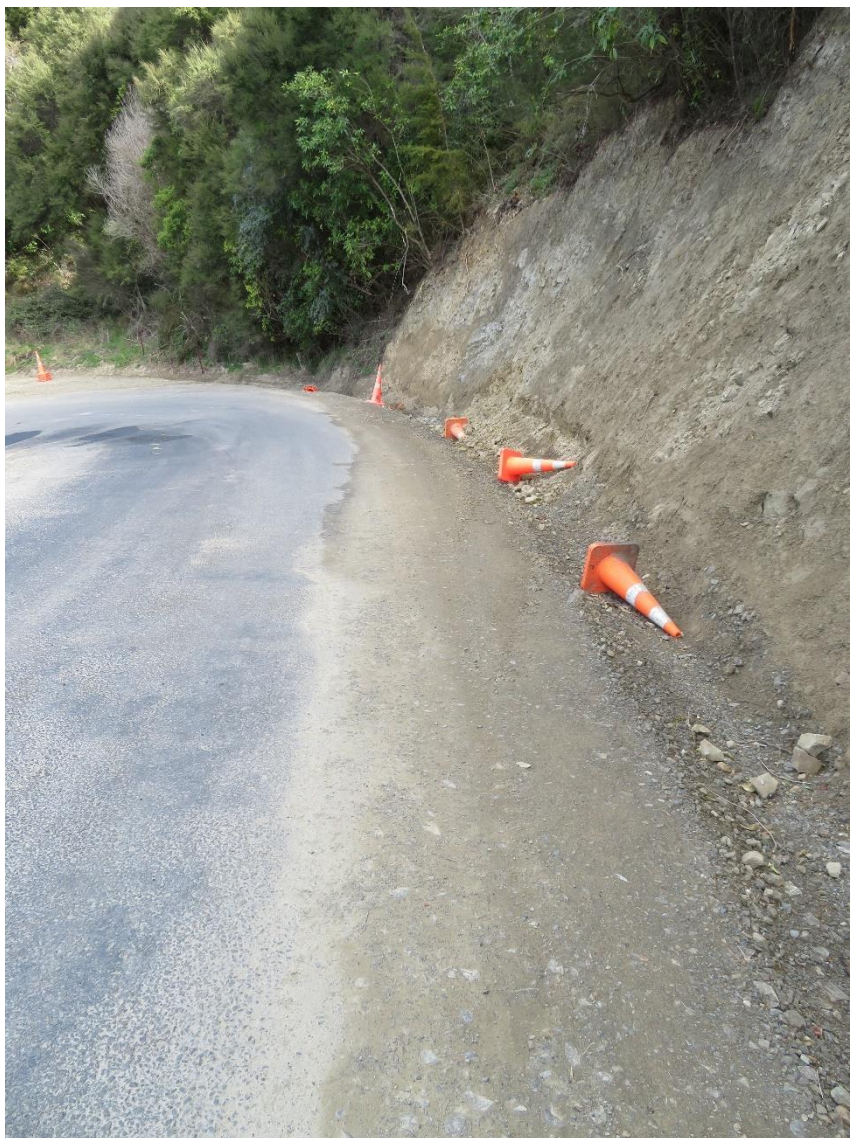
Photo 4: Waireka Road staircase switchback improvements by Wairoa District Council.
