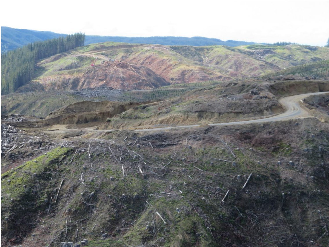
Photo 1: Looking at Landing 24 operations from Aropaoanui Road.
