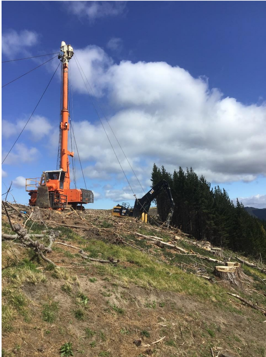
Photo 5: Setting up hauler for two-stage operation on Setting 3A to Setting 3.
