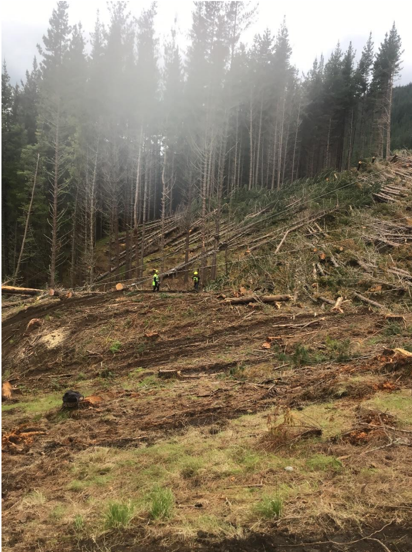
Photo 10: Log 2 breaker outs discussing drag selection due to limited lift because of rimrock bluffs.
