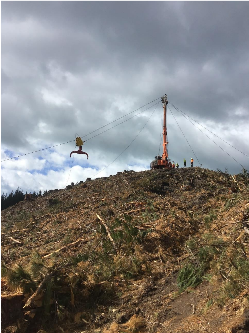
Photo 7: Log 2 running the new acme claw out for the first drag.
