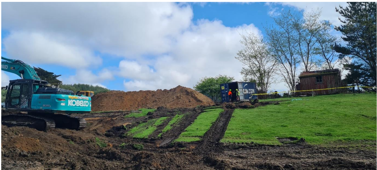
Photos 1, 2 & 3: Beginning of entrance through paddock into forest and protected historic building.
