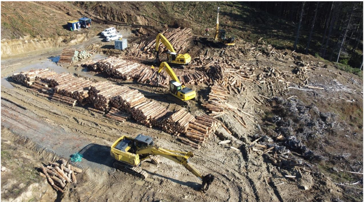
Aerial view of Landing 138 showing log stacks sorted nicely for loadout.
