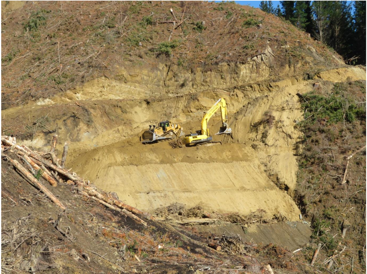
Photo 1: Large bench for construction of McCoy Road.
