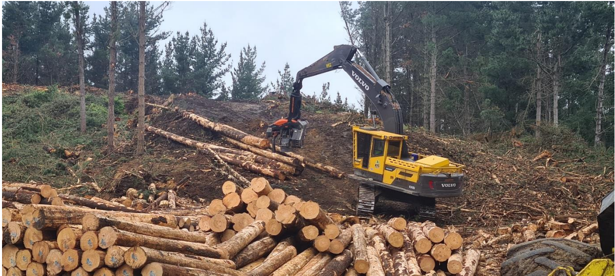
Photo 1: Felling machine on Landing 31.
