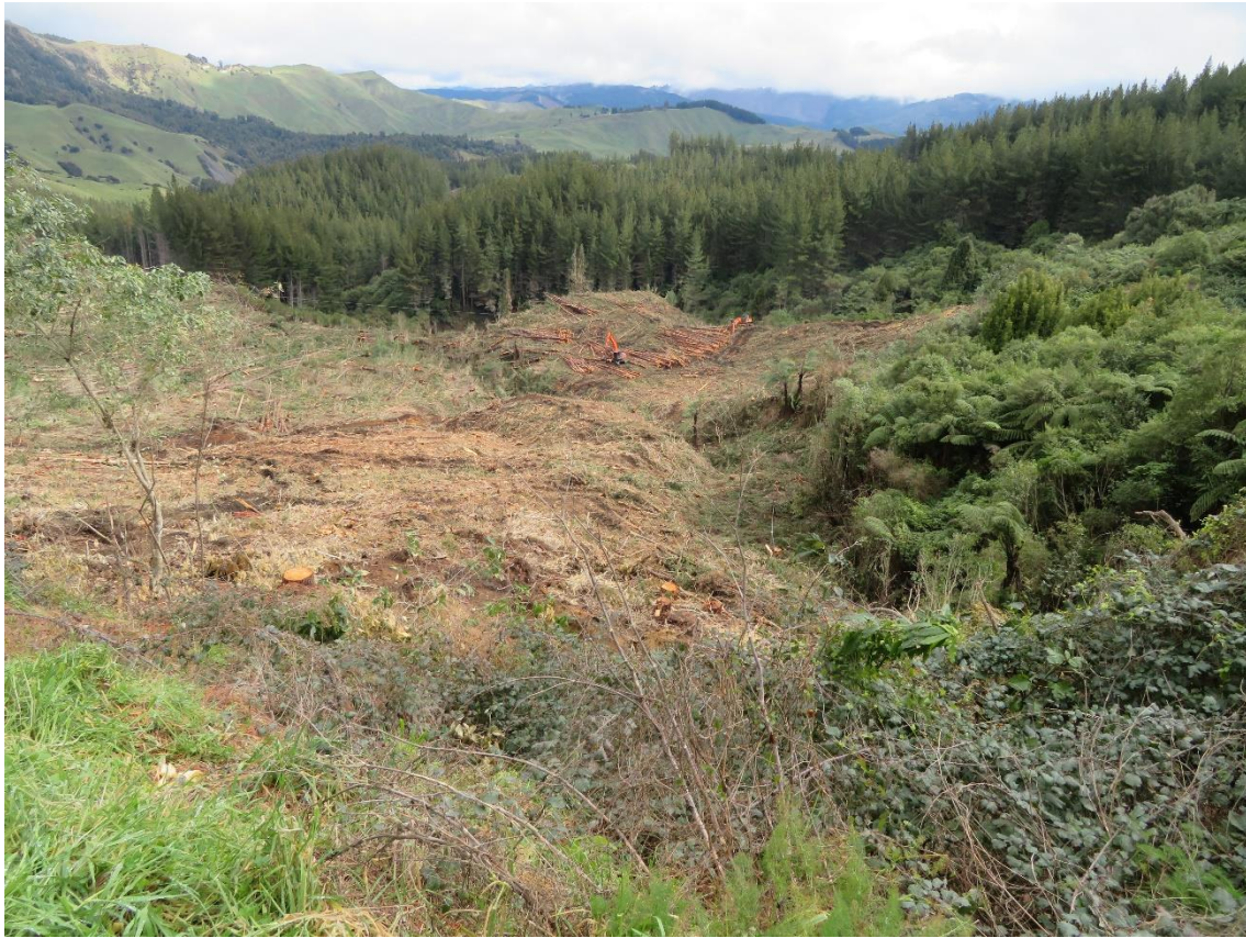
Photo 1: Setting 65, shovelling the backline.
