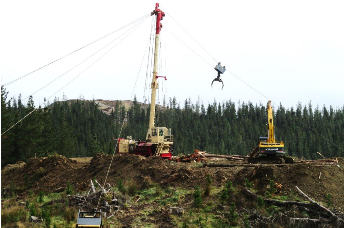
Photo 2: Log 11 hauler at Pad 18A.
